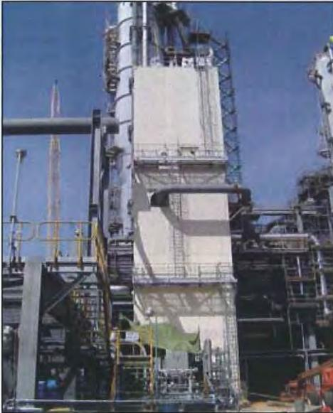
KBR proprietary cryogenic purification technology removes methane, argon and excess nitrogen from synthesis gas and allows use of air instead of oxygen in the reforming section of the ammonia plant, eliminating the need for an expensive air separation unit.
