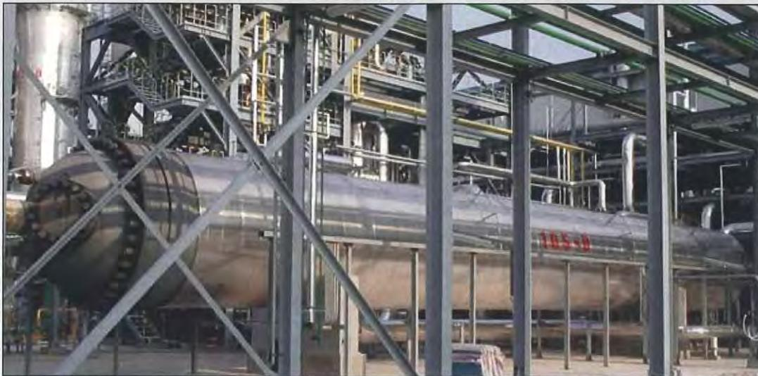
For conventional magnetic ammonia synthesis loops, KBR offers its horizontal ammonia synthesis converter. Inner-stage coolers between the catalyst beds provide for maximum conversion and heat recovery.
