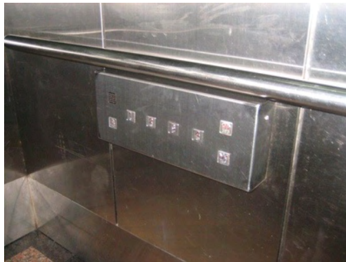
Photo 2-5-5 KL Sentral Station elevator (1)
