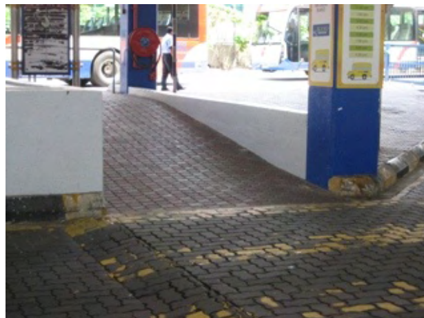
Photo 2-5-11 Bus terminal slope (Kelana Jaya)
