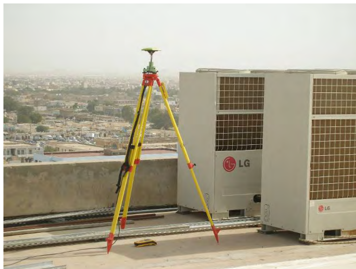
Figure 2.14 La station de base
