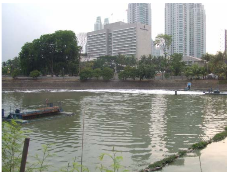
Picture 3.3.1 Setiabudi Aerated Ponds
