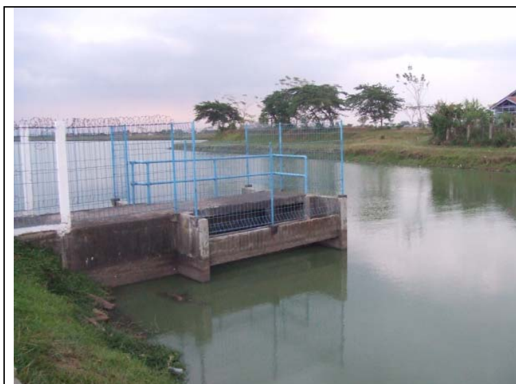
Picture 4.3.7 Bojongsoang WWTP
