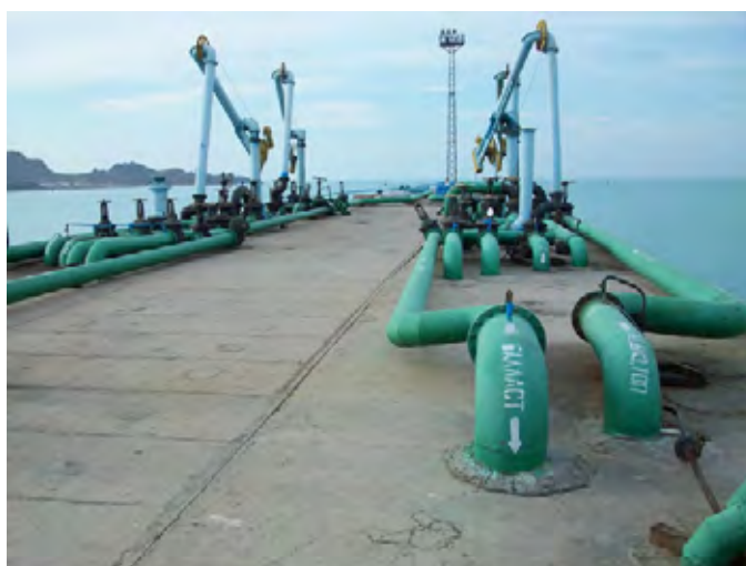
Figure 2.1.29 PPK3 UFRA Terminal (South Jetty)
