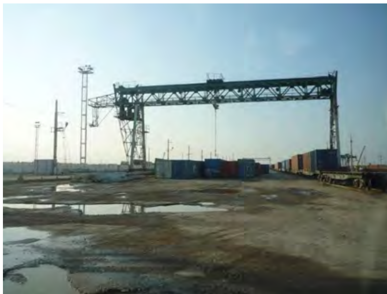
Gypjak Container Station
