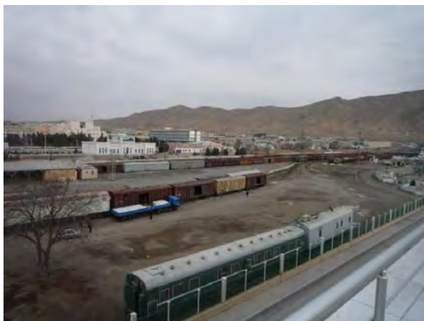
Transshipment Facilities between Railway and Truck at Turkmenbashi
