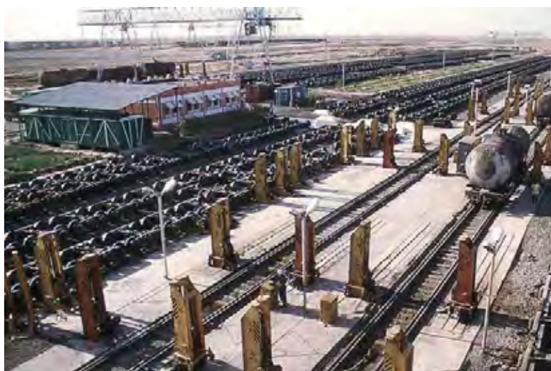
Bogie Exchange Facilities, Serakhs
