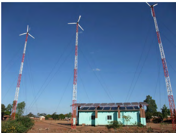
Photo 5 Solar village (Wind & PV) Wind towers are located in front of PV array that cause shade during daytime.
