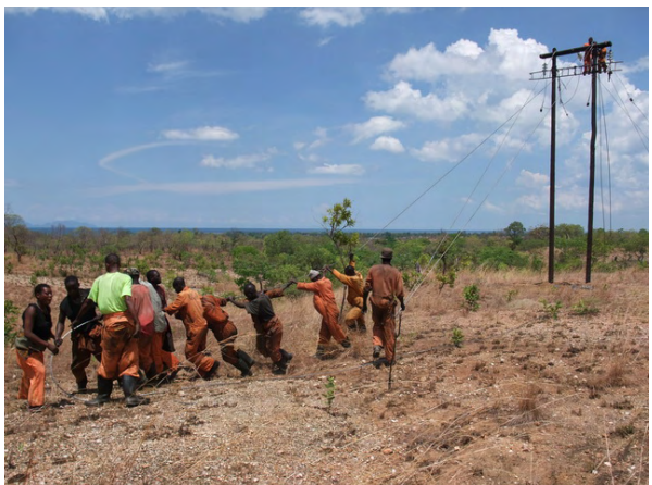
Photo 6 Construction at Makanjira
