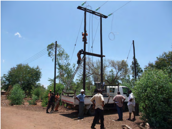
Photo 7 Construction at Makanjira
