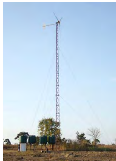
Photo 5: A wind irrigation system by UNDP (No functioning due to no wind)
