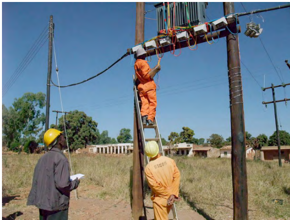
Photo 3 Inspection by ESCOM
