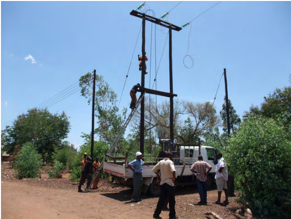
Photo 7 Construction at Makanjira
