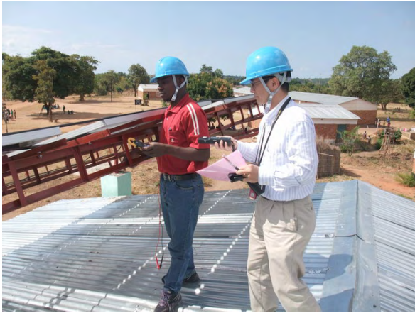
Photo 7 Inspection of PV array
