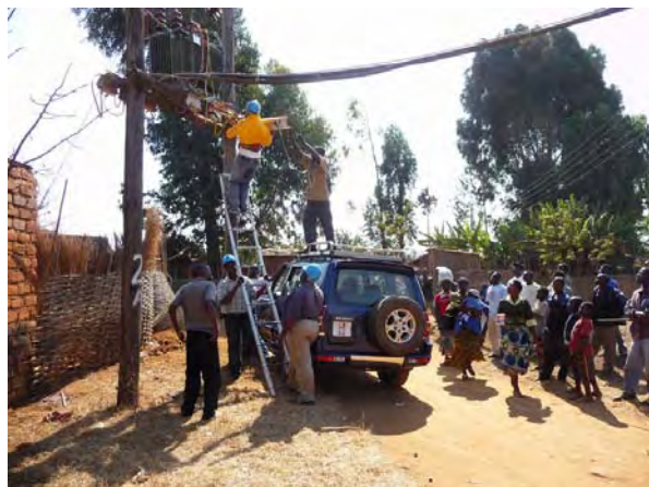
Photo 2 Installing data logger at the transformer
