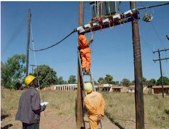
Photo 3 Inspection by ESCOM
