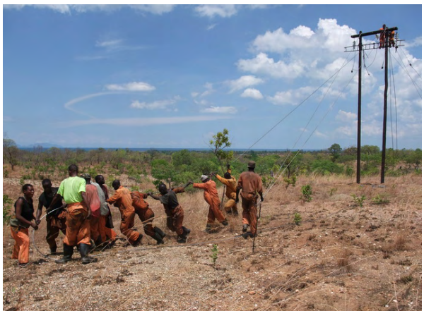
Photo 6 Construction at Makanjira
