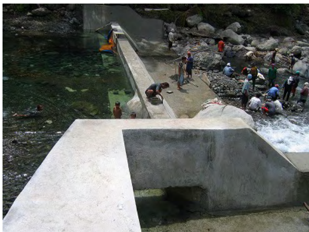
Completed Intake Weir
