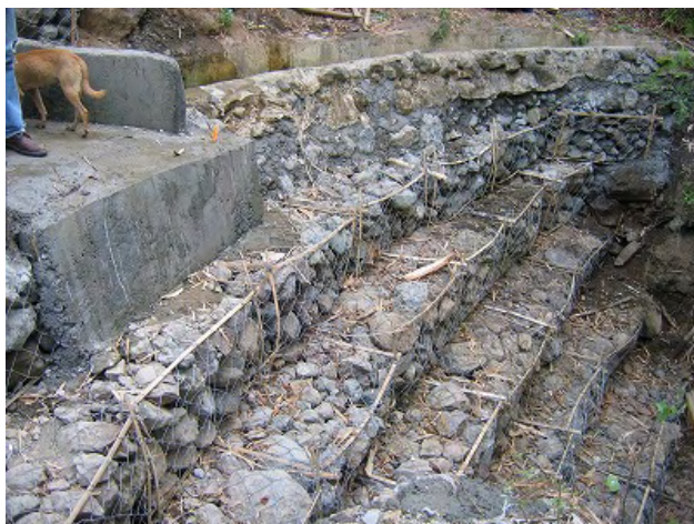
Gabion Installation
