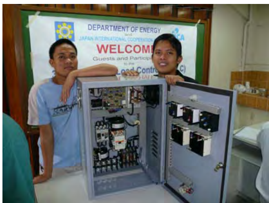
Completed ELC Box
