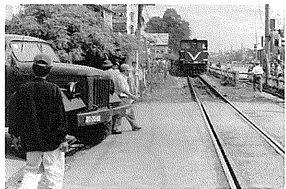
Non -existence of a barrier at level-crossing
