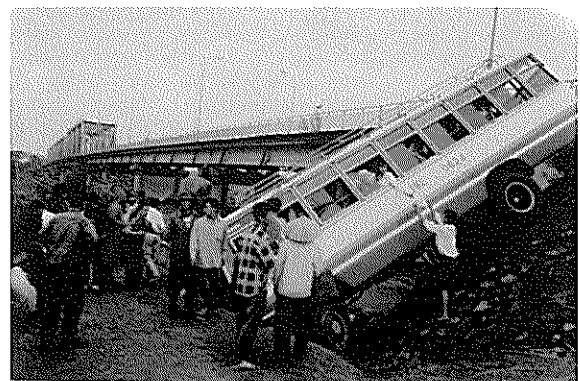
An accident at Phong Chau bridge in Phu Tho province
