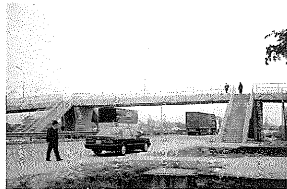
Pedestrian flyover on National Road No.5
