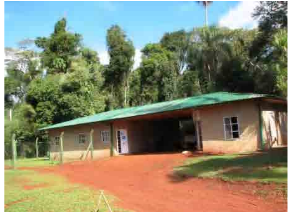
Photo 2. Yacuy office built by the Project, Iguazu National Park near the East border entrance
