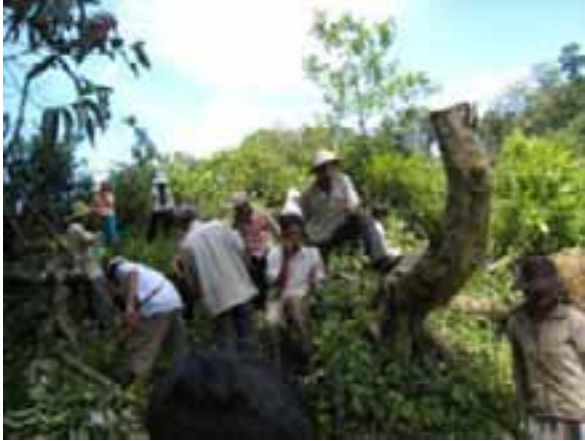
Clearing vegetation and hole digging
