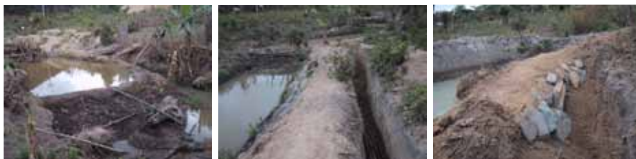
Pond making works (February 2008)
