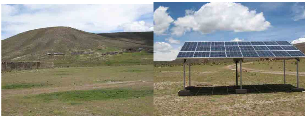
Figure IV-1 Centro poblado of Vilcallamas (left) and solar panel (right)
