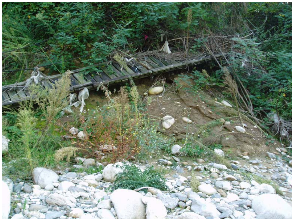
Figure B.2.1 Damaged Hydrometric Station
