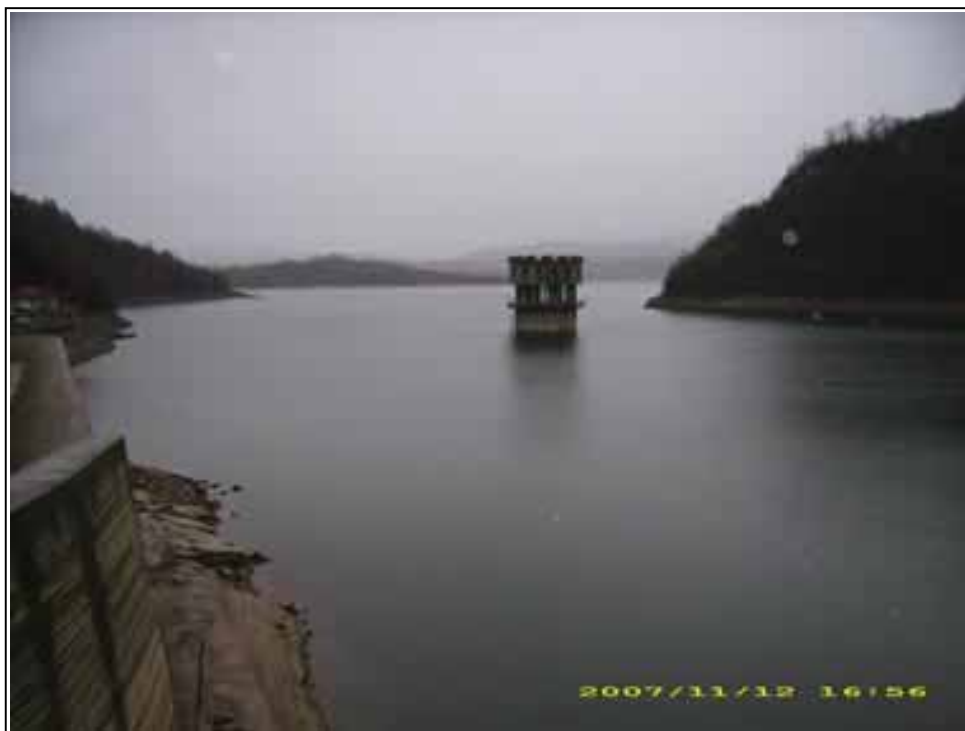
Pic.9 – Tower intake of Yovkovtsi reservoir
