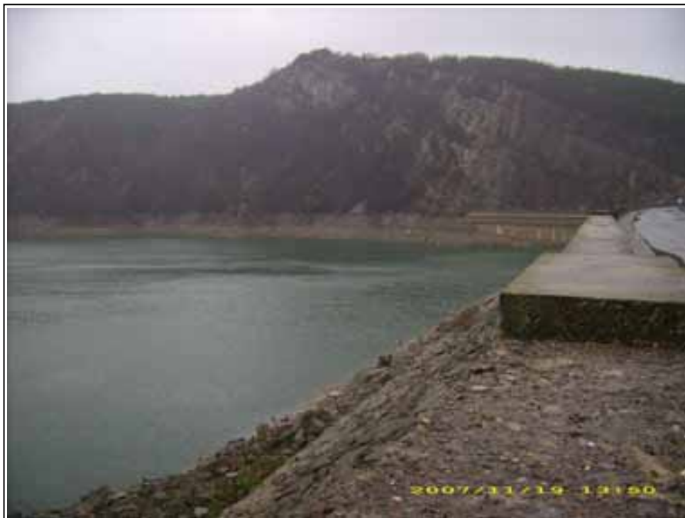
Pic.1 – General view of Kamchia reservoir and rockfill dam
