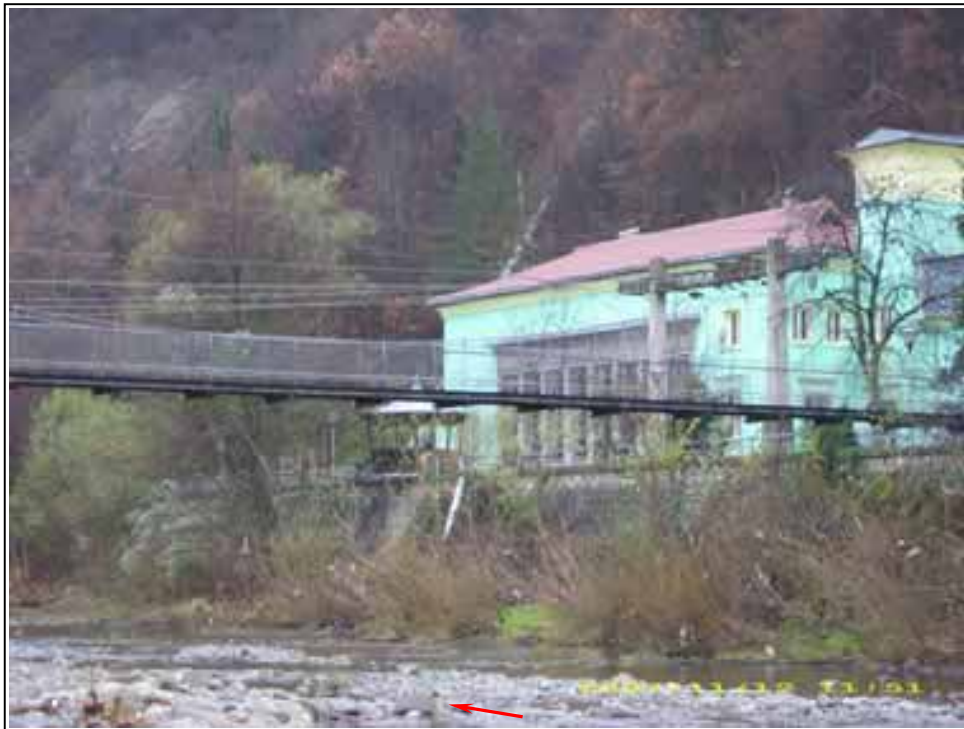
Pic.5 – Batoshevo-1 HPP at Batoshevo village on the Rositsa River
