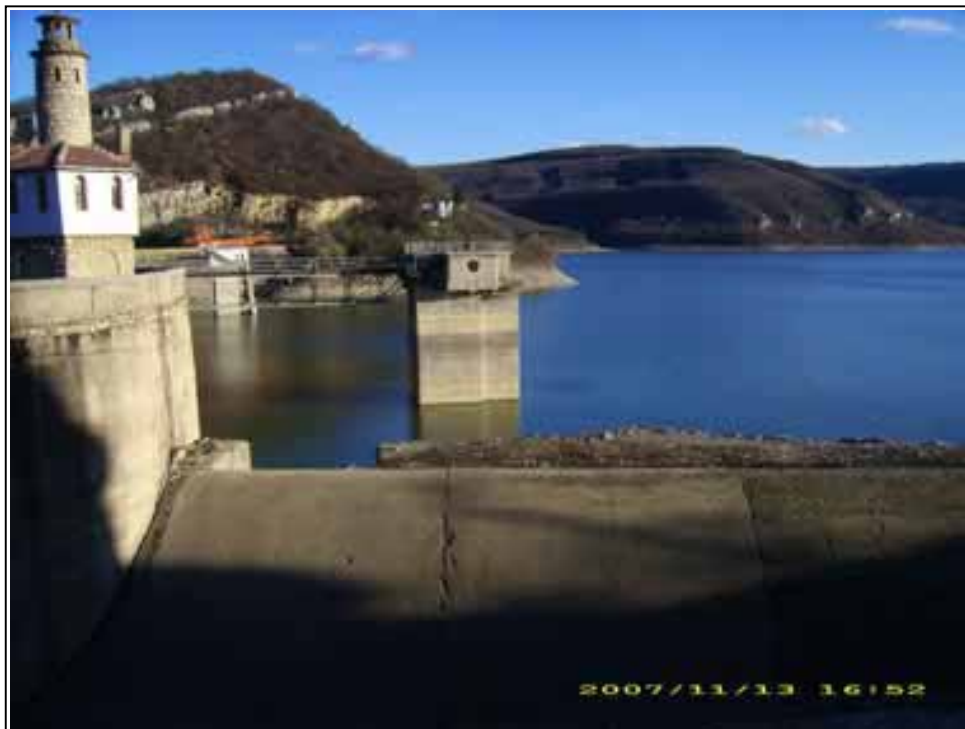
Pic.21 - General view of Alexander Stamboliiski reservoir, dam and tower intake
