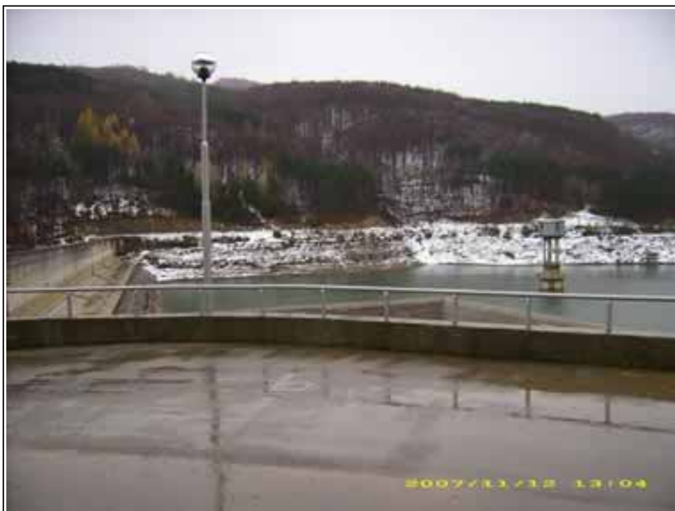
Pic.6 – General view of Hristo Smiranski reservoir, dam and tower intake
