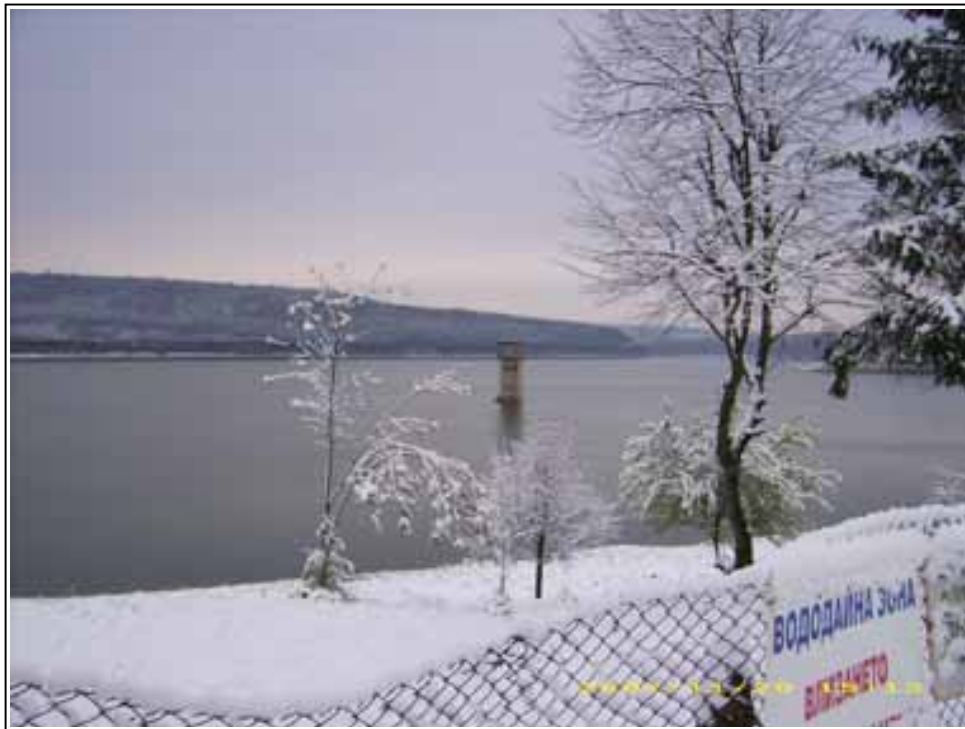
Pic.13 - Ticha reservoir and tower intake
