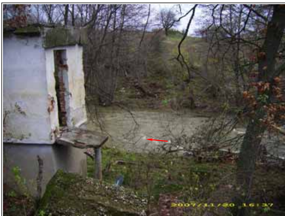
Pic.16 - Abandoned HMS No.43500 and destroyed observation hut at Beronovo village on the Luda Kamchia River
