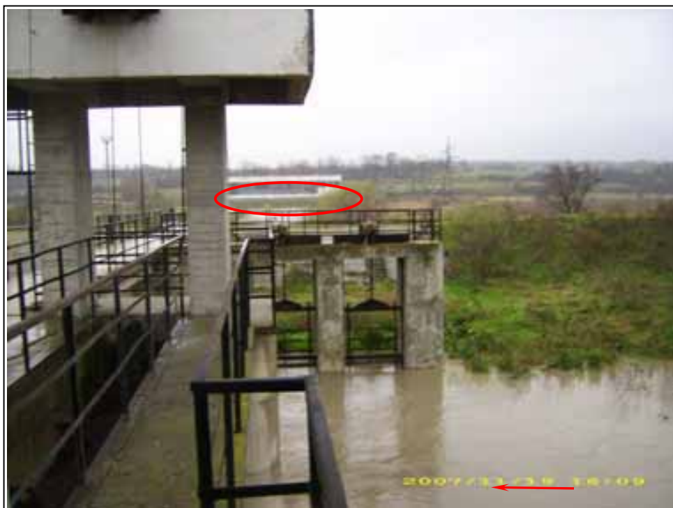
Pic.4 – Detailed view of the gate mechanism, flooded irrigation intake and lifting pump station (red circle) behind the water pool
