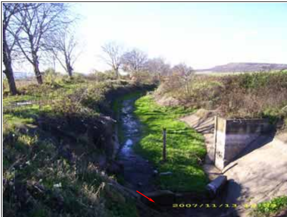
Pic.17 - Nikyup irrigation channel at Lesicheri village on the road bridge
