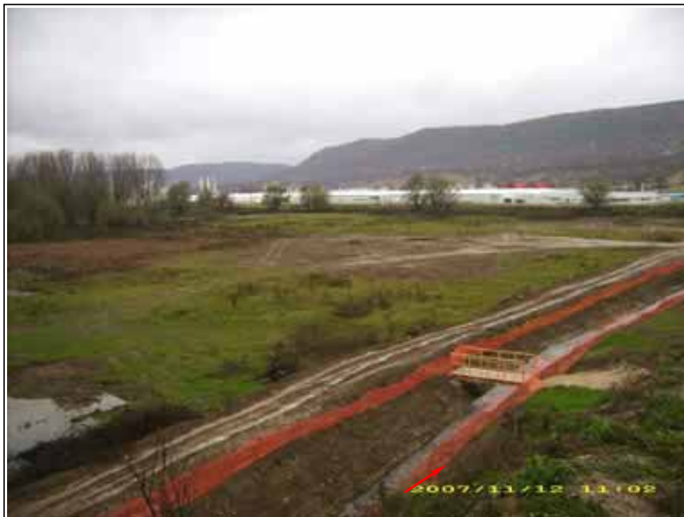
Pic.1 – General view of Sevlievo WWTP construction site
