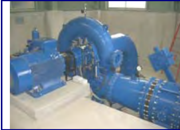
ກົງຫັນລິເວີສປ໌ (Reversible Pump Turbine (Nam Mong 70 kW))
