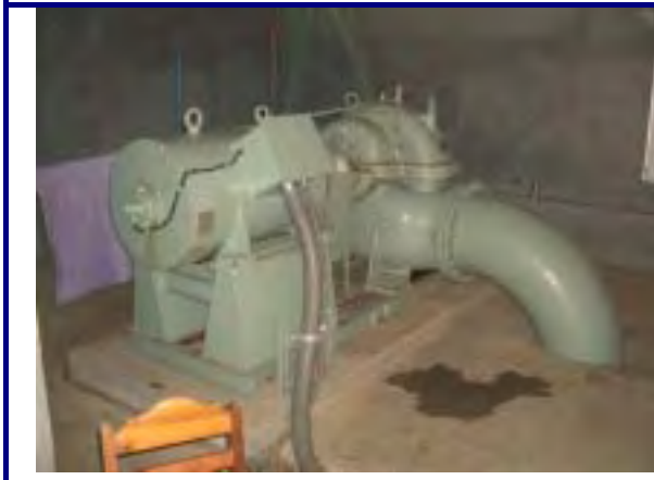
ກົງຫັນລິເວີສປ໌ (Reversible Pump Turbine (Nam Mong 70 kW))
