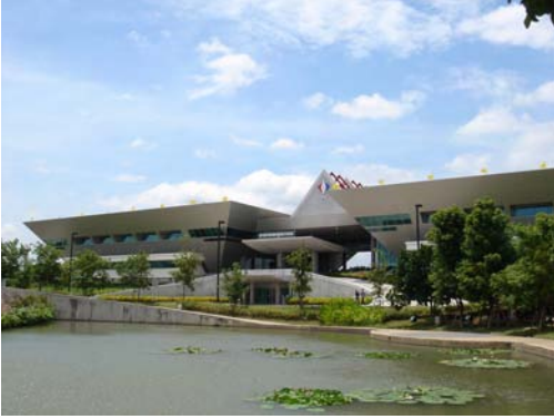
New NIMT Building
