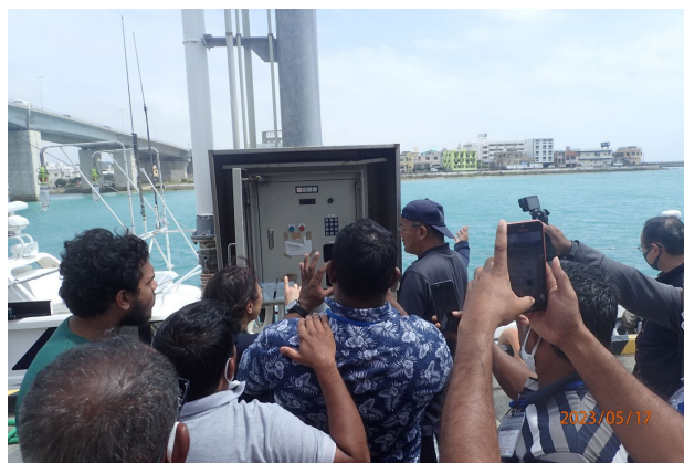
Photo 8-4 Facilities of Itoman FCR
