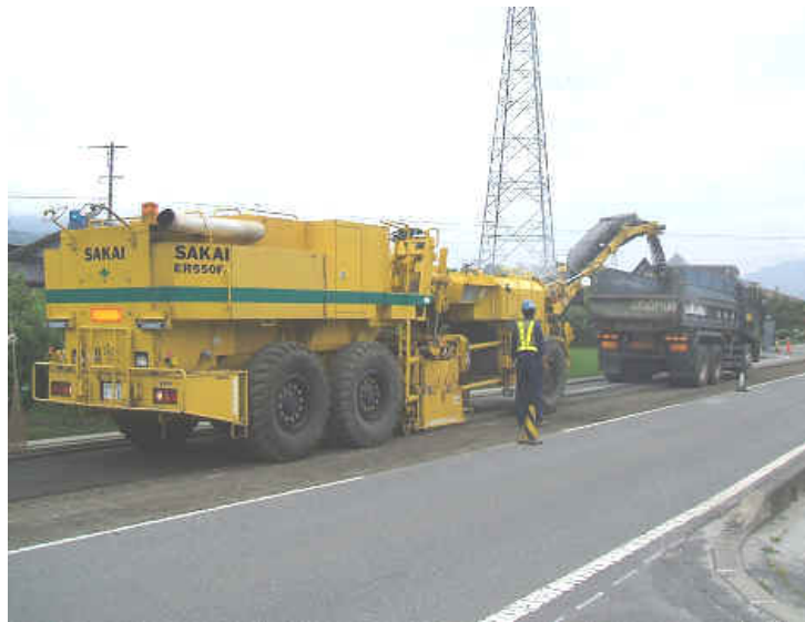
Figure 80 Road Surface Cutting by Road Surface Milling Machine
