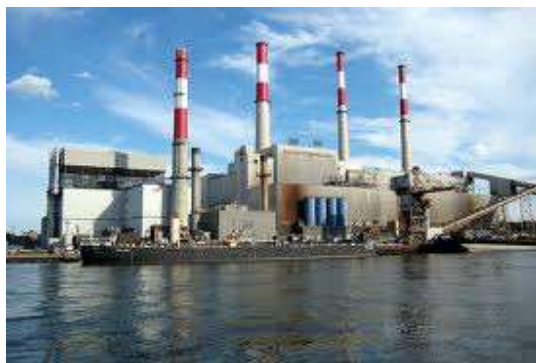
Figure 1.3. Egbin Thermal generating unit.
