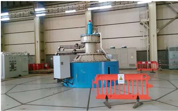
Figure 1.4. Refurbished 1G6 (120MW) at Kainji
