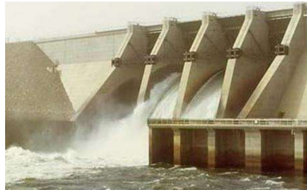
Figure 1.5. Kainji Hydro Spill Gate.
