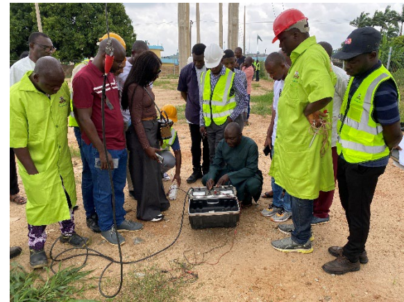
NAPTIN Practical Training Demonstration (Overhead Line Fault Location) (10th July, 2025)
