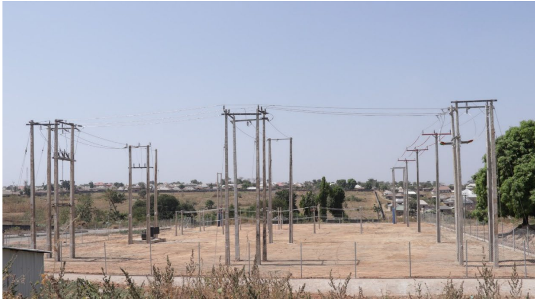
Figure 2-1-2.2 Full View of Distribution Training Facilities
