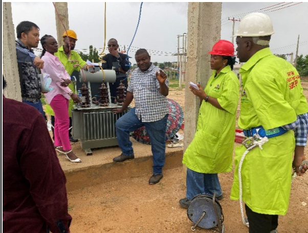
TOT on Overhead Line Fault Location at NAPTIN (Lecturers dispatched from AEDC) (29th June, 2025)
