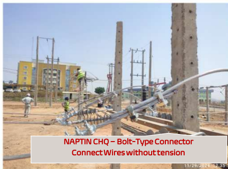
NAPTIN CHQ - Conductor Cover Prevent contact with obstacles
