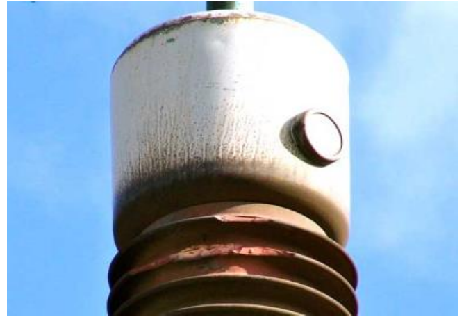
Figure 9 Chipped and Rusted Porcelain
