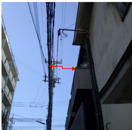
Figure 11 Structures too close to Distribution Tower
