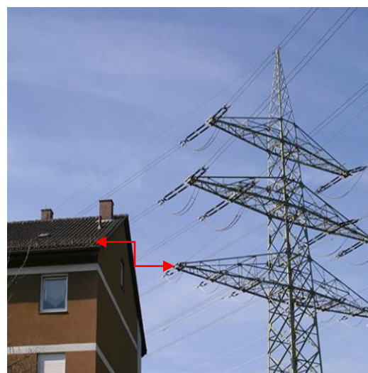
Figure 11 Structures too close to Distribution Tower
