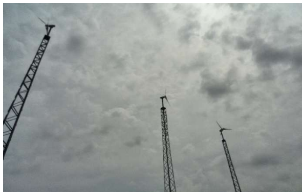
Figure 1.7. 15kW Wind Plant at Kainji
