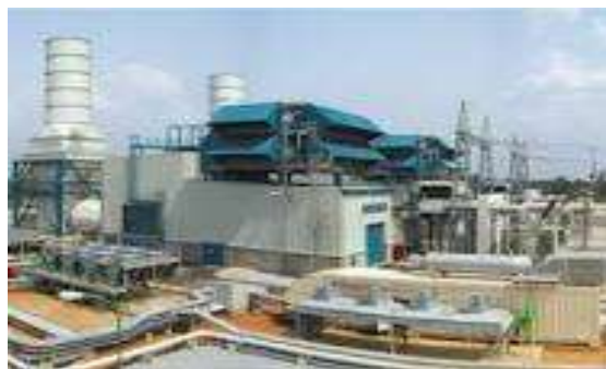
Figure 1.8. Afam VI Gas Power Plant.
