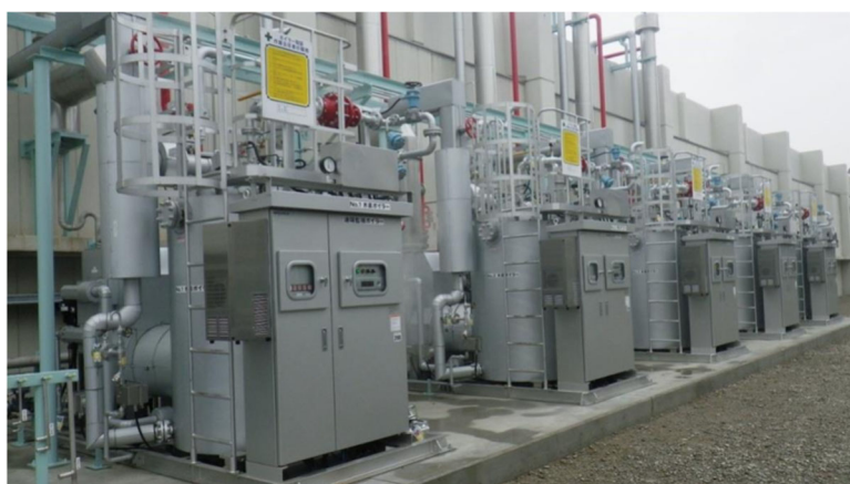
Figure 5-34 Hydrogen Boiler Facilities implemented in Chemical Plant
