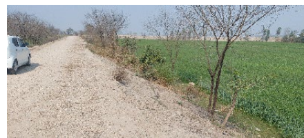
Facing Upstream Side
