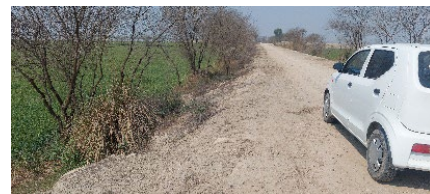
Facing Upstream Side
