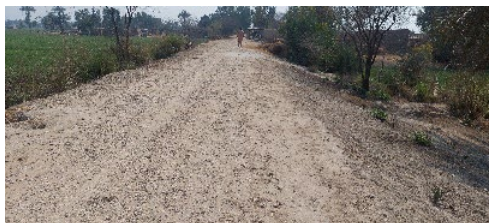
Facing Downstream Side
