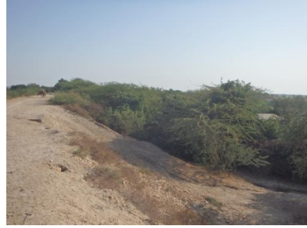
Facing Upstream Side
