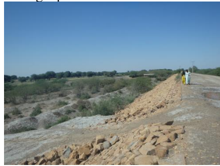
Facing Upstream Side
