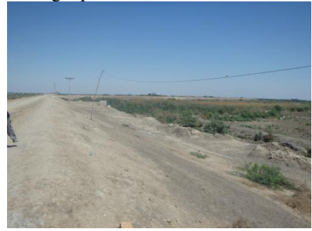
Facing Upstream Side
