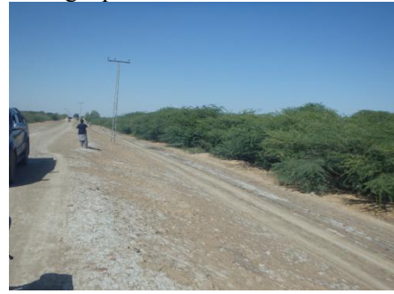
Facing Upstream Side
