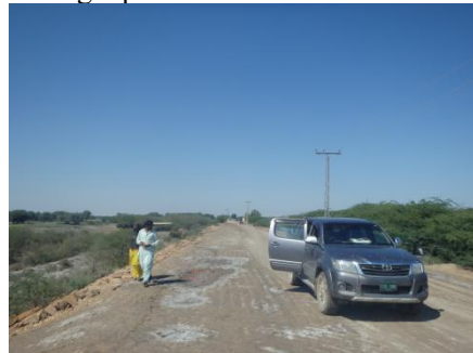
Facing Upstream Side
