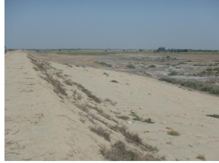
Facing Upstream Side
