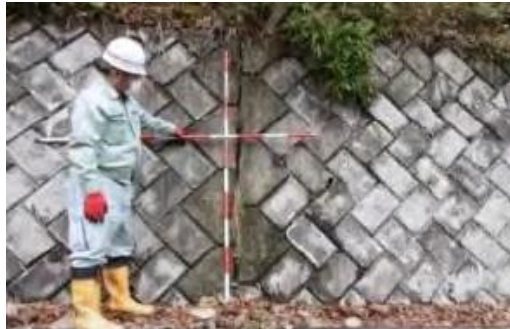
Concrete block masonry wall (Leaning type)
