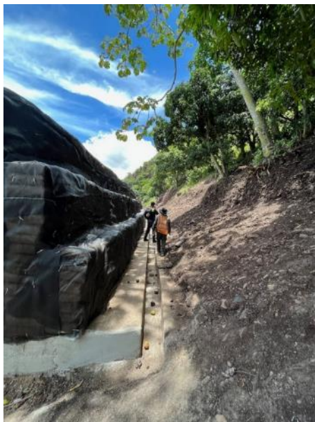
Figure 81 Case study of rockfall protection wall in Honduras (Fuerzas Unidas)
