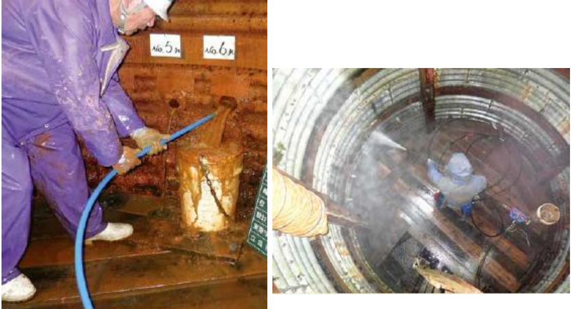
Figure 39 Cleaning situation (Case of horizontal drainage boring in well)
