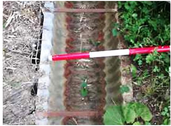
Rust in steel channel
