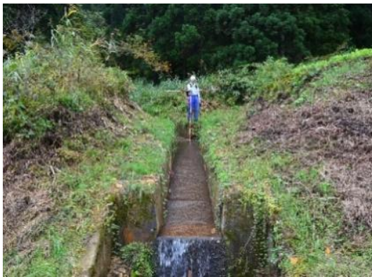
Surface water control work (Channel work)
