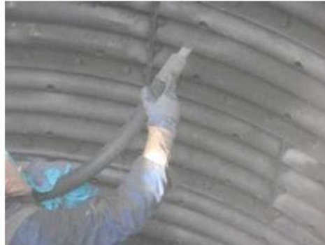
Sandblasting (Removal of rust)
