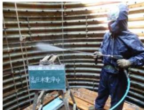
Cleaning surface of wall material
