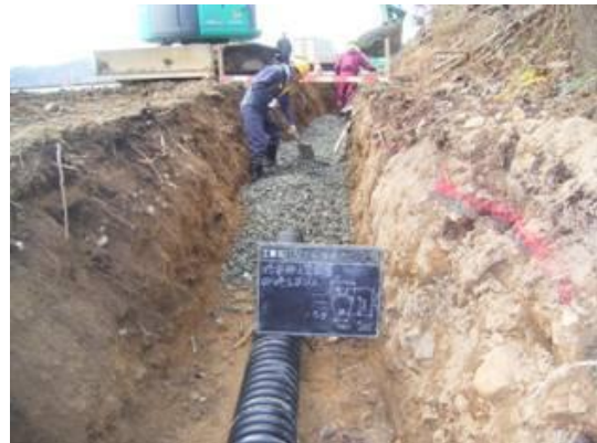
Shallow ground water control work (Drain work)
