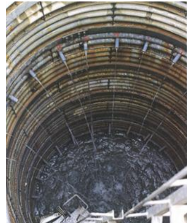
In side of drainage well
