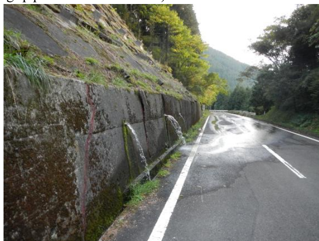
Large amount of spring water
