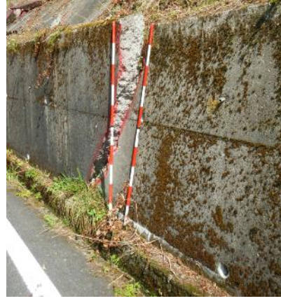
Retaining wall is broken and tilted by landslide activity.
