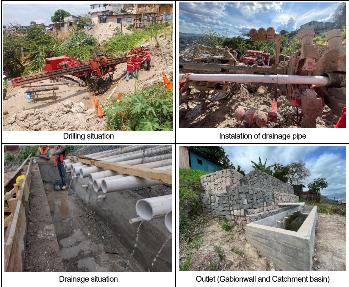
Figure 13 Case study photos of Horizontal drainage boring (In Campo Cielo)
