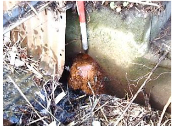
Blockage of drainage pipe outlet due to slime
