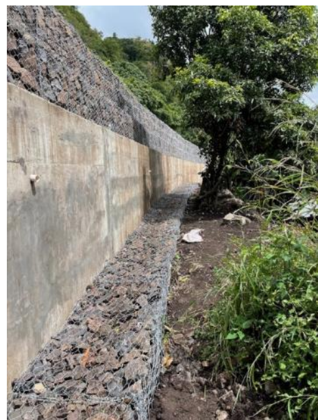
Figure 81 Case study of rockfall protection wall in Honduras (Fuerzas Unidas)
