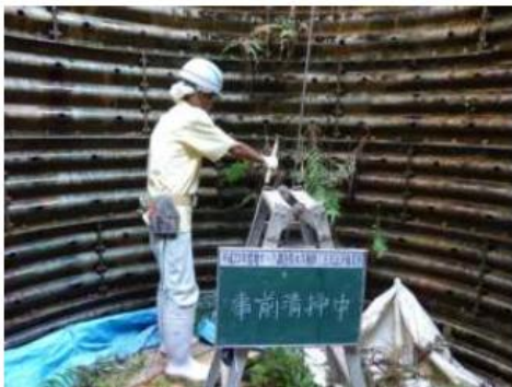
Removal of vegetation and sediment
