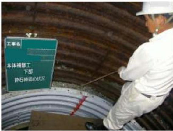
Filling crushed stone behind inner liner plate
