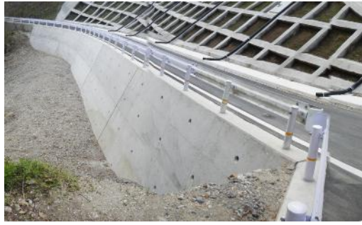
Concrete retaining wall (Gravity type)
