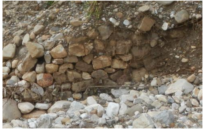
Collapsed gabion
