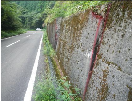
Retaining wall is broken and tilted by landslide activity.
