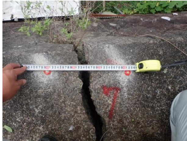
Figure 30 Crack monitoring (Measuring markings or rivets)
