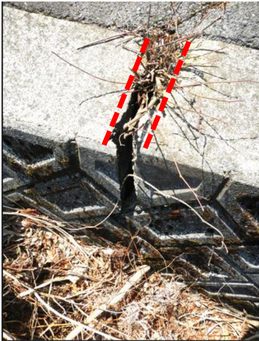
Retaining wall shift between joints by landslide activity
