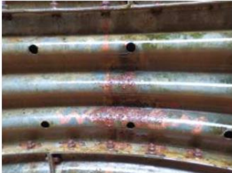
Situation of surface after cleaning
