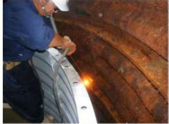
Install inner liner plate
