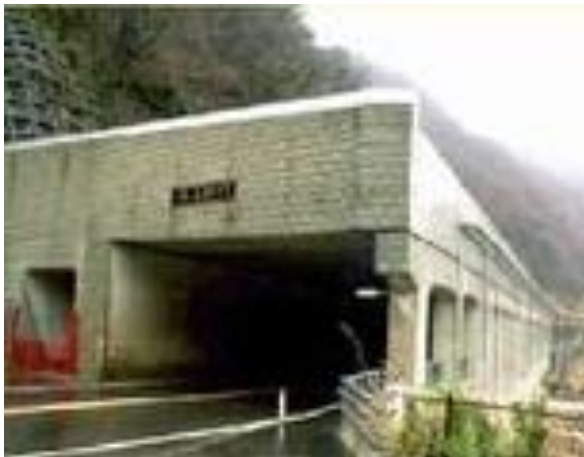
Figure 82 Case study of rock shed in Japan
