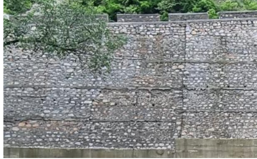
Stone wet masonry wall (Gravity type)
