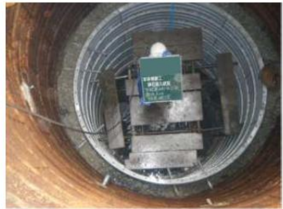
Extend pipe of horizontal drainage boring
