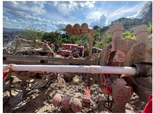
Drainage pipe installation
