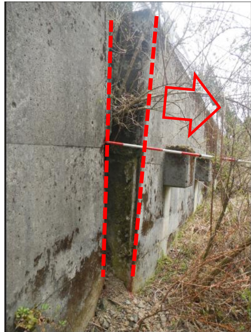
Retaining wall shift between joints by landslide activity
