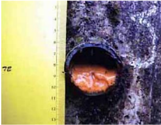
Blockage of drainage pipe outlet due to slime
