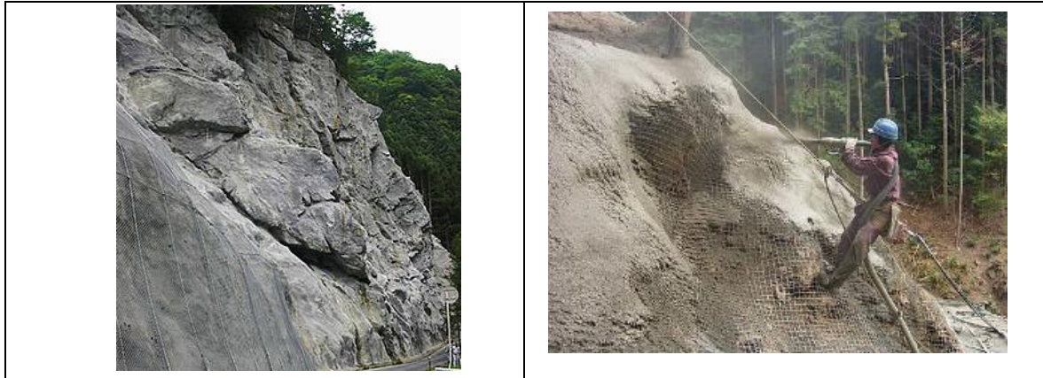
Figure 35 Case study photos of shotcrete work
