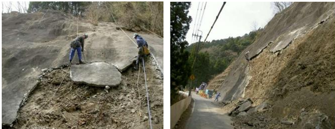
Figure 61 Manual demolition situation
