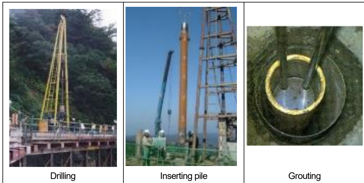
Figure 29 Pile construction situation
