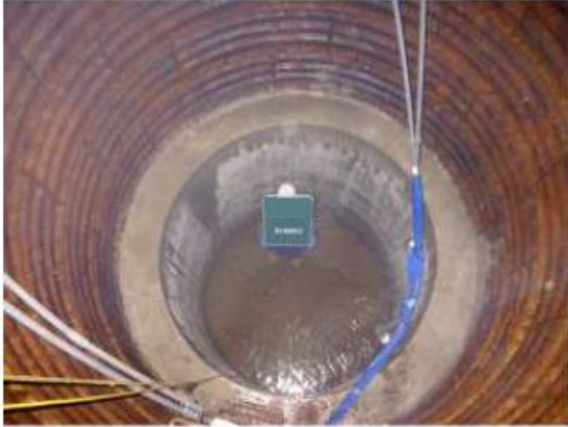
Thickening concrete of catchment basin
