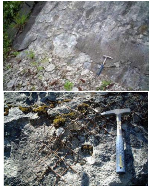
Figure 24 Image drawing and case study photo of peeling
