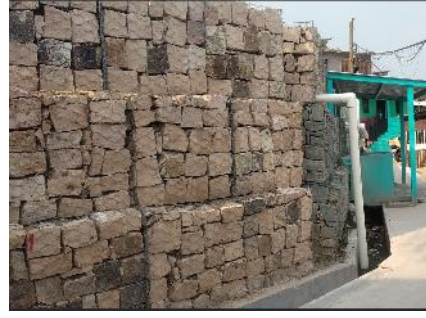
Gabion retaining wall (Leaning type)
