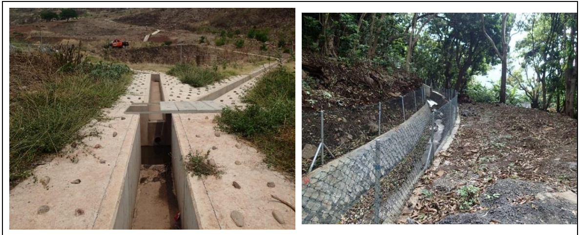
Figure 1.34 Surface Drainage System in Landslides (JET)
