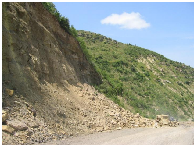
Figure 0.4 Slope Failure (JET)
