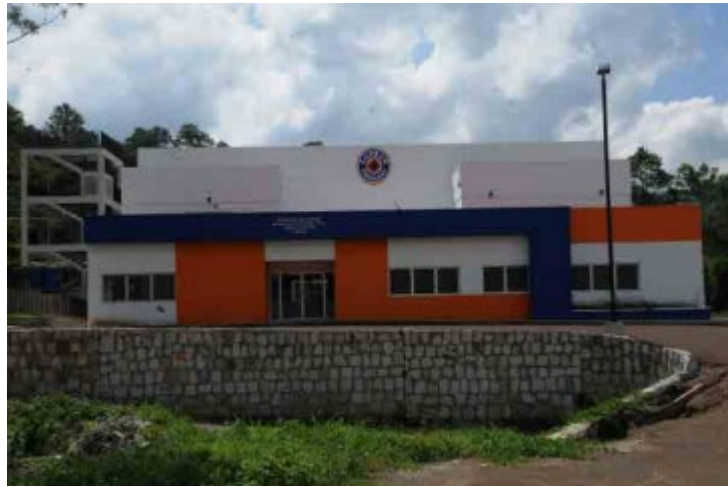
Figure 85. COPECO Training Centre. (Source: COPECO)
