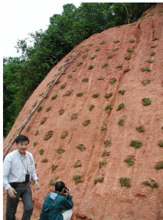
Figure 2.21 Simple Vegetation Works in Malaysia
