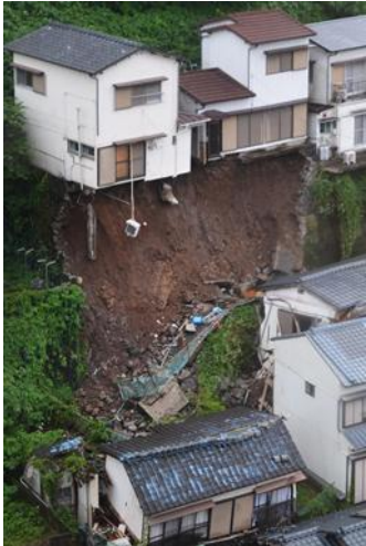
Figure 2.16 Houses above /under Steep Slope Collapsed (The Mainichi)
