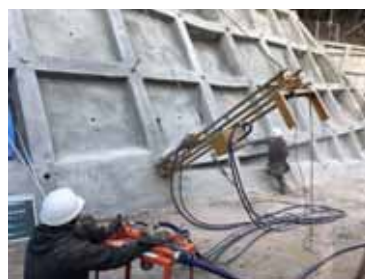
Drilling by boring machine
