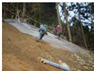
Wire mesh installation
