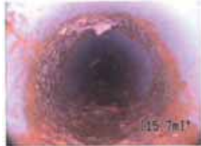
Clogging of drain pipe due to slime
