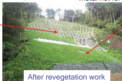
Vegetation base material spraying work
