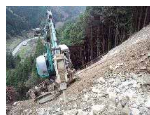
Excavation with hanging excavator
