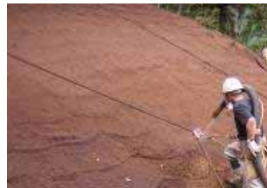
Vegetation base material spraying work
