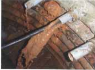
Cleaning of holes with high-pressure water
