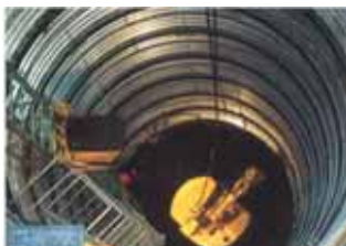
Drainage well excavating situation
