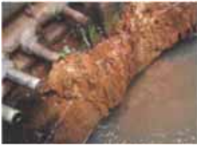
Clogging of drain pipe due to slime
