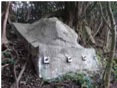
Foot protection work
