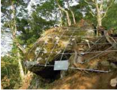
Rope net setting work
