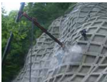
Crane hanging drilling method
