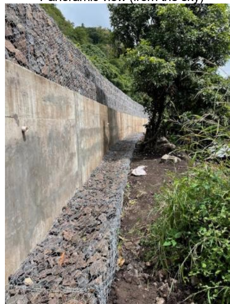
Gabion, foundation concrete
