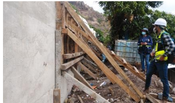
Setting form work situation
