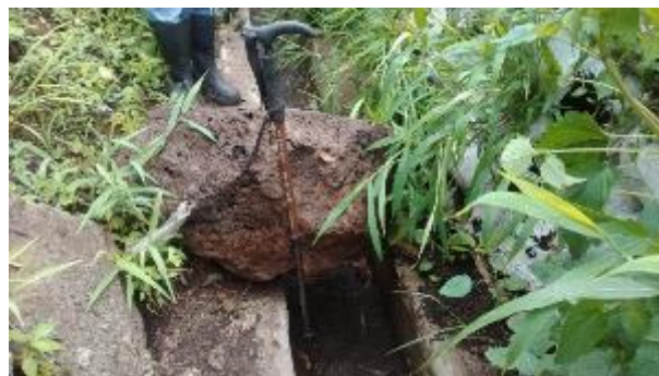
Figure 144 Falling rock captured situation
