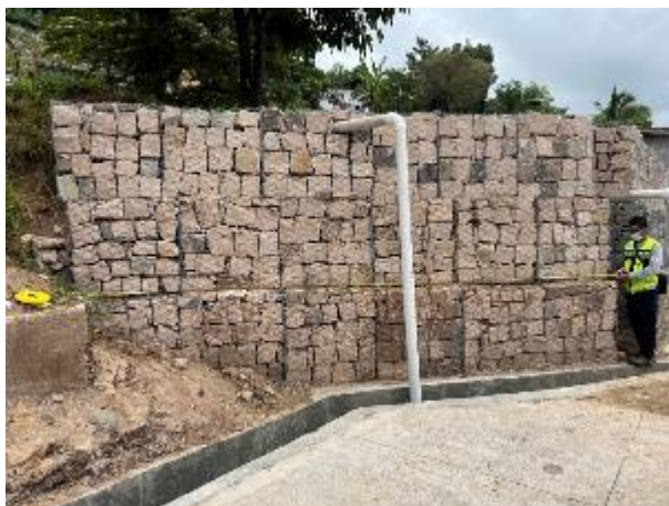
Retaining wall length measuring situation
