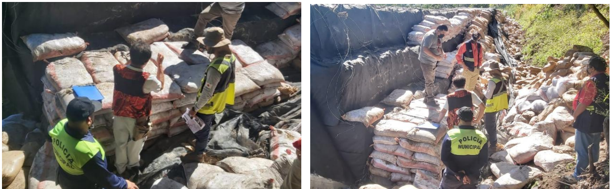
Figure 141 Sandbag repair work guidance and consultation situation
