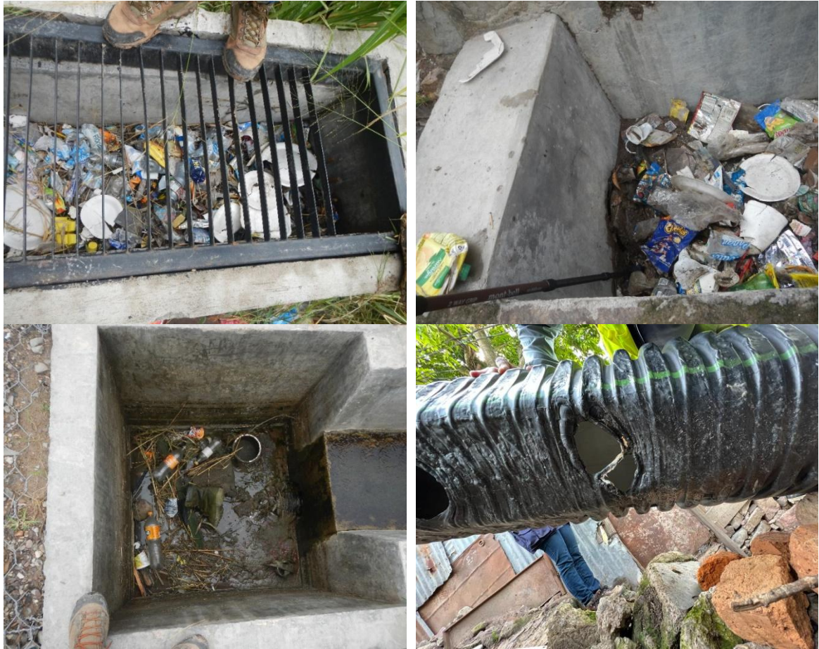
Figure 139 Current facility situation
