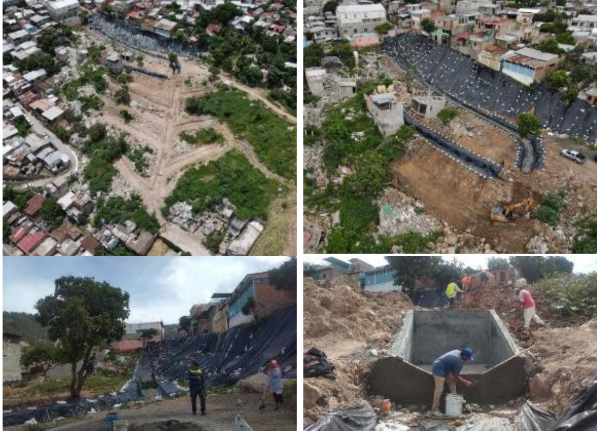
Figure 130 Construction situation of emergency countermeasure
