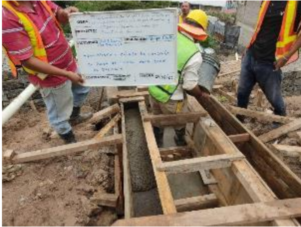
Channel construction situation
