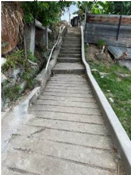
Water stop concrete
