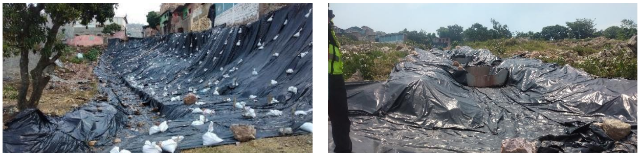
Figure 146 Monitoring and maintenance situation (May 2024)
