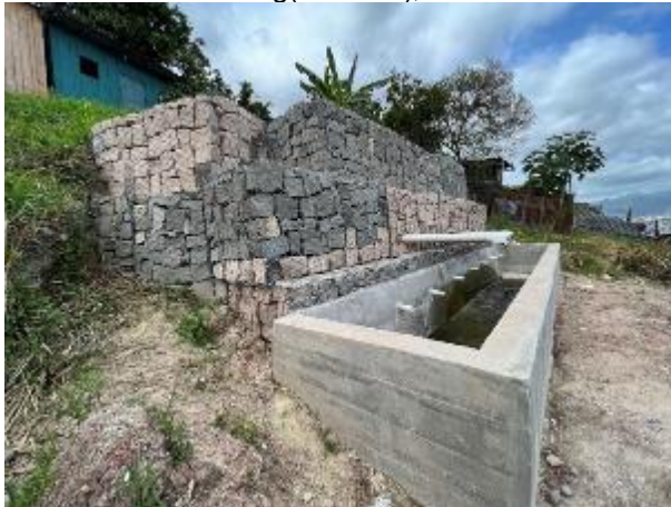
Horizontal drainage boring(Section3), Catchment basin
