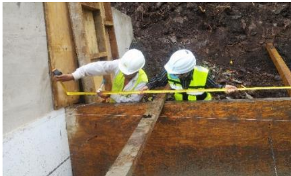
Measuring form work situation
