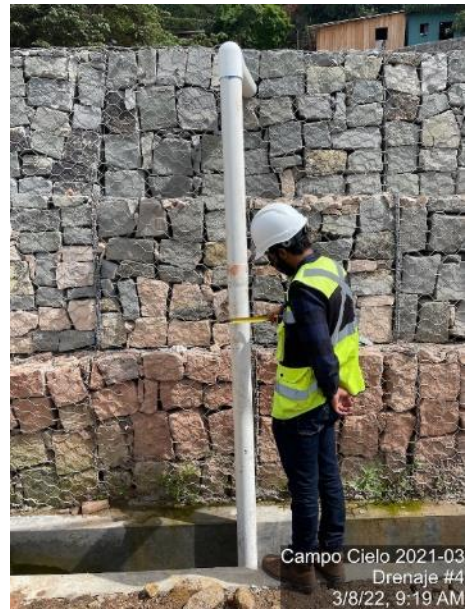
Horizontal drainage boring dimension measurement situation
