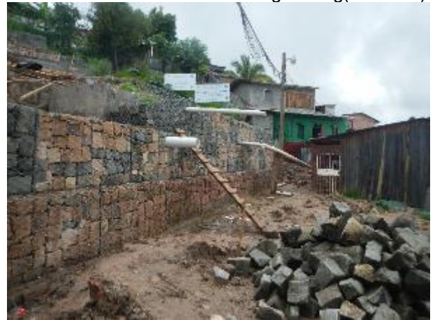
Retaining wall construction situation
