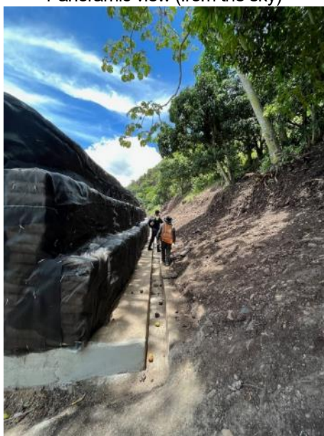
Sandbag stack, Gutter
