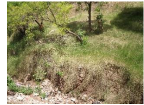
Scouring riverbed/ bent trees at roots.
