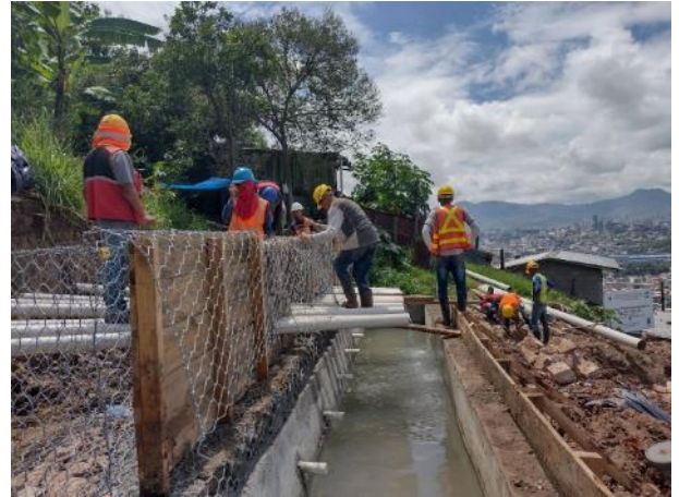
Catiment basin of horizontal drainage boring(Section 3)
