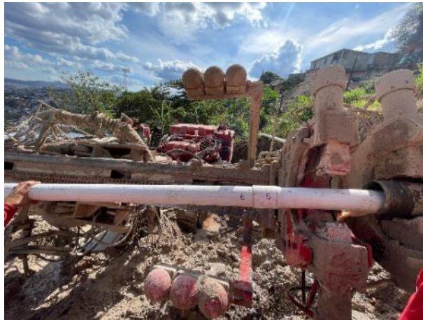
Install drainage pipe
