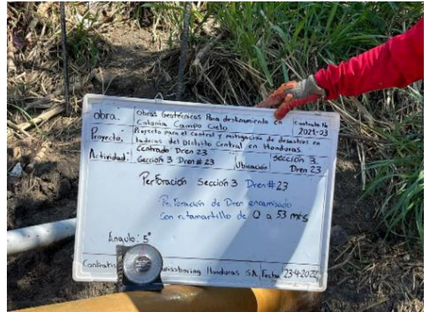
Drilling angle checking situation
