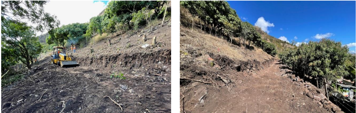
Figure 118 Progress of the construction works in Fuerzas Unidas
