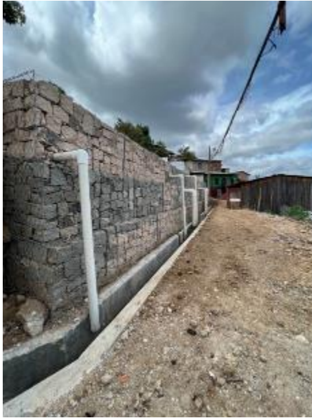
Retaining wall, Horizontal drainage boring(Section1), Gutter
