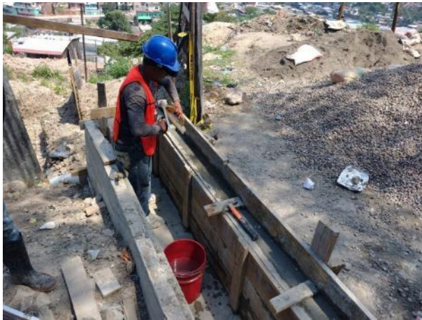
No.2Gutter construction situation
