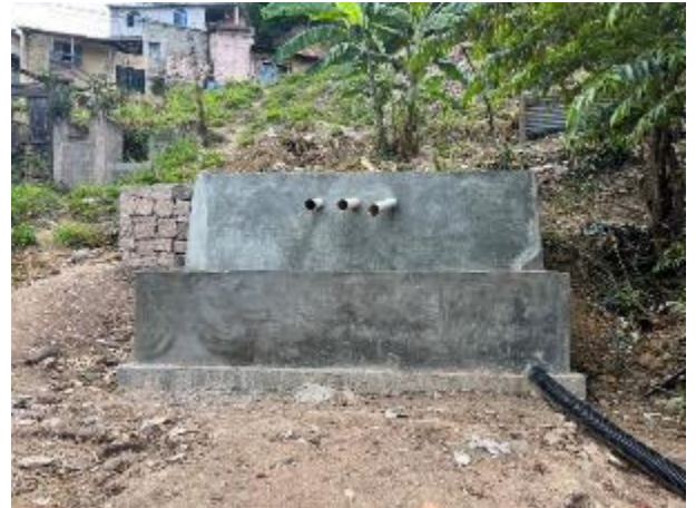
Horizontal drainage boring(Section2), Catchment basin
