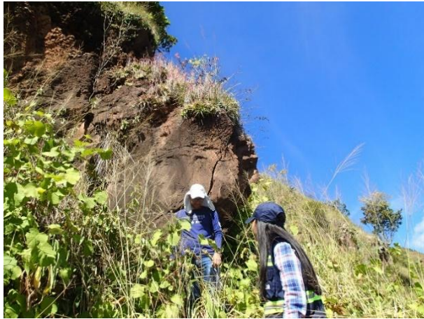
Figure 16 Unstable rock survey
