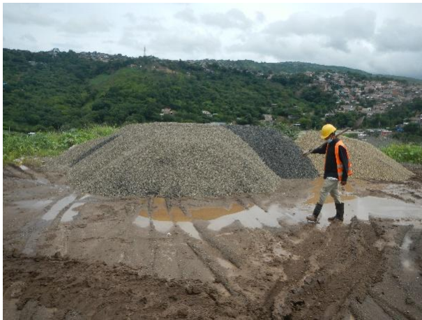
Coarse aggregate storage condition
