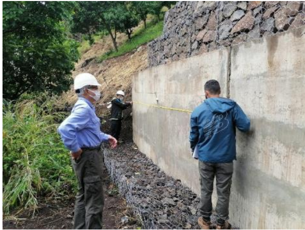
Foundation concrete dimensions measuring situation
