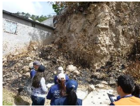
Vertical opening crack
