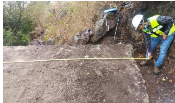
Measuring concrete foundation sizesituation
