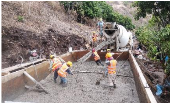
Placing concrete situation
