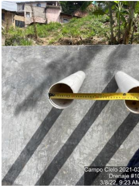
Horizontal drainage boring dimension measurement situation
