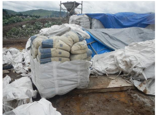
Cement storage condition
