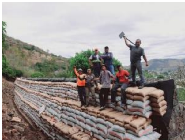
Figure 143 Sandbag repairing completion situation
