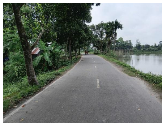
Paved Upazila Road (Non-Submersible) – Asphalt Pavement, Width: 5.5 m
