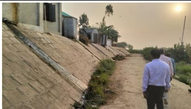
Village Protection Walls (Kishoreganj District)
