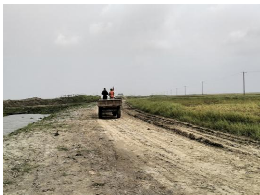
Unpaved Upazila Road (Submersible) – Requires Improvement
