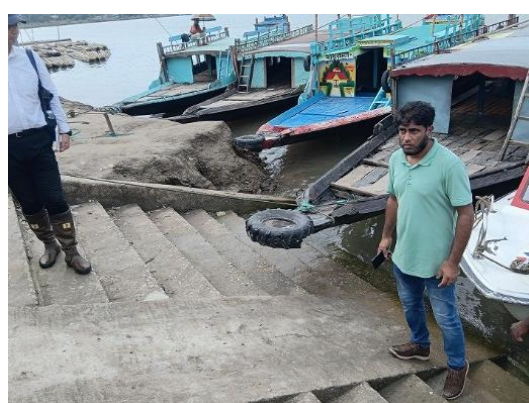
Existing Boat Landing Stations (Reinforced Concrete Structures, Approximately 5.0 meters in Width)
