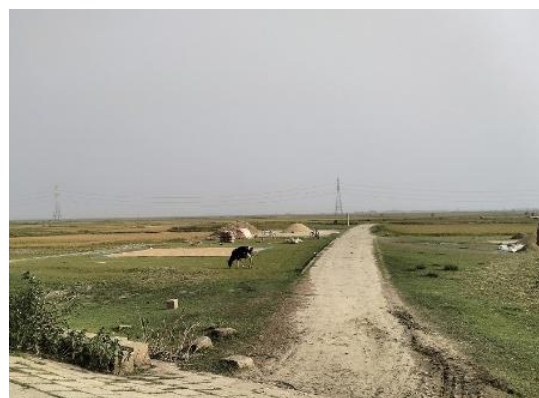
Village Road (Submersible) – Condition during Non-Submersion (Reinforced Concrete Pavement, Road Constructed under Phase 1)
