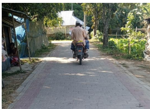
Example of Uni-block Pavement Construction by LGED (Mymensingh Office)
