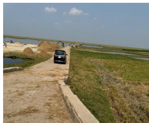
Union Road (Submersible) – Condition during Non-Submersion (Reinforced Concrete Pavement, Carriageway Width: 3.0 m)
