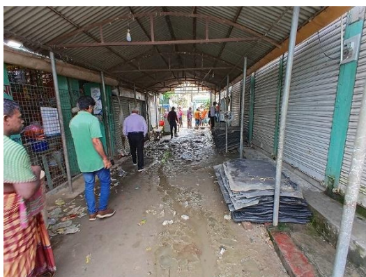
Existing Growth Centers (with Roofing, but Lacking Adequate Paving and Drainage Facilities)
