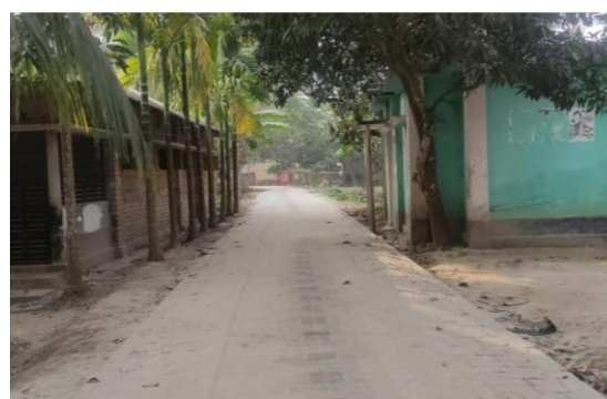
Example of Uni-block Pavement Construction by LGED (Rajshahi Office)
