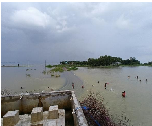
Village Road (Submersible) – Condition during Submersion (Reinforced Concrete Pavement)
