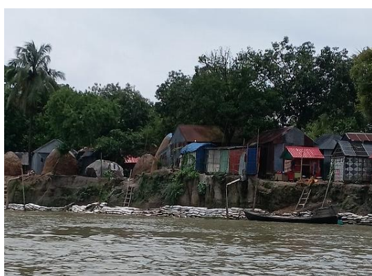
Village Protection Walls Constructed by the Villagers Themselves (Defenses using Sandbags and Vegetation)
