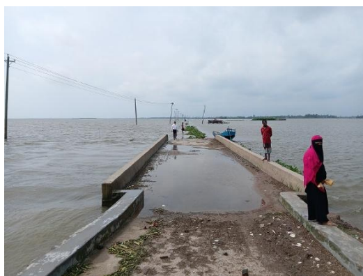
Union Road (Submersible) – Condition during Submersion (Reinforced Concrete Pavement, Carriageway Width: 3.0 m)
