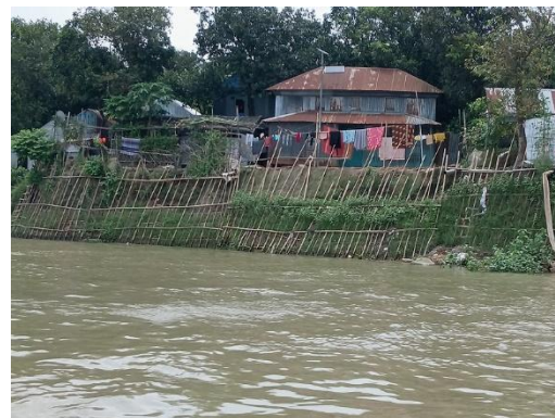
Village Protection Walls Constructed by the Villagers Themselves (Defenses Consisting of Wooden Fences and Vegetation)
