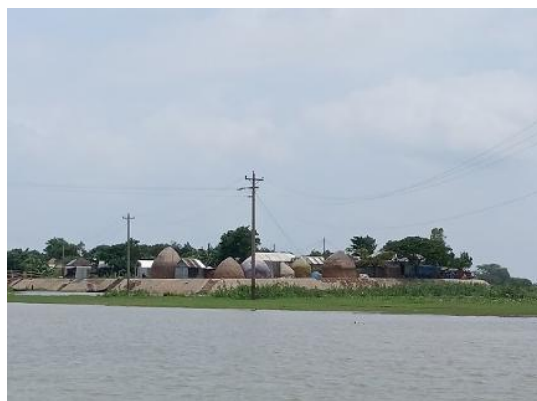
Village Protection Walls Constructed under other Donor Projects (Bank Protection using CC Blocks, HILIP)
