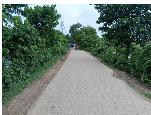
Paved Union Road (Non-Submersible) – Condition (Asphalt Pavement)
