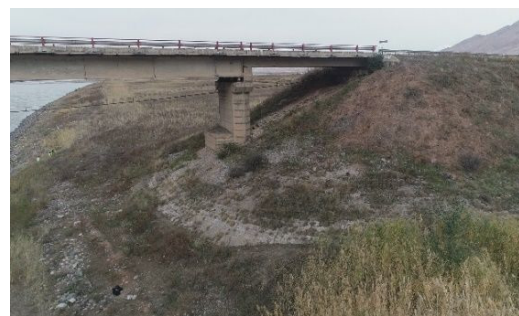
Panoramic view: Right bank revetment
