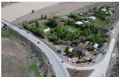
Photo 1-2-7 Settlement south of the project site
