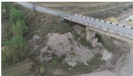
Panoramic view: Left bank revetment
