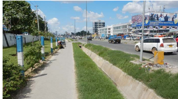
Sidewalk and Trapezoidal Open Ditch
