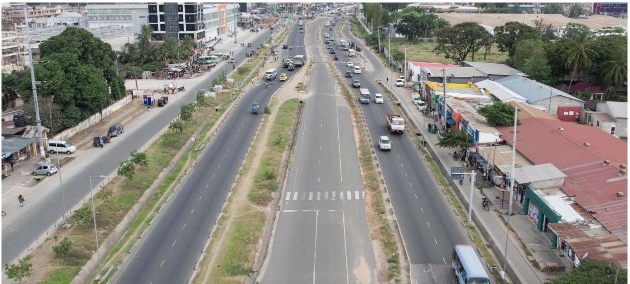
Construction of BRT Station (Mwenge / ITV Station) is planned.
