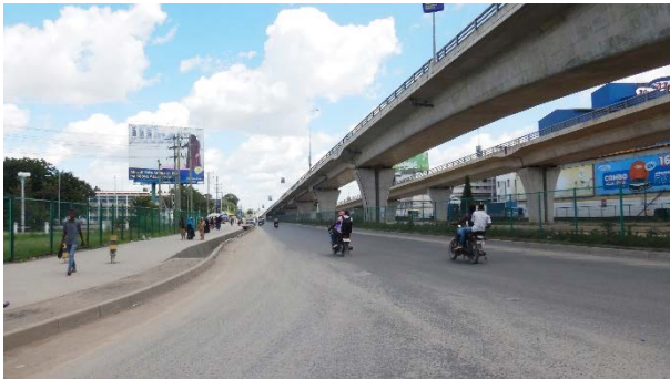
Outbound Lanes to Airport Side
