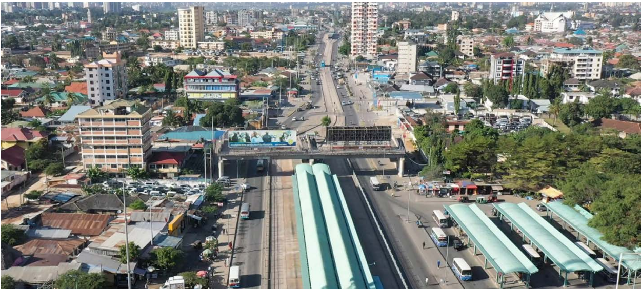
Pedestrian Bridge for Accessing BRT Station
