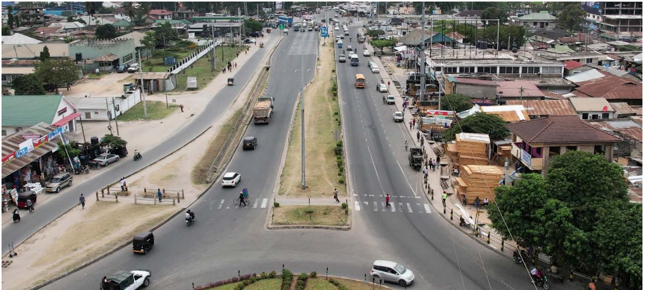
Construction of BRT Terminal Station (Mwenge Terminal) is planned.
