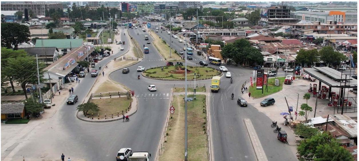
Roundabout with TRA Road
