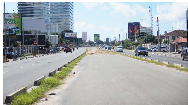
Center Median for BRT corridor
