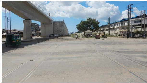
SGR Viaduct and at-grade Railway Crossing
