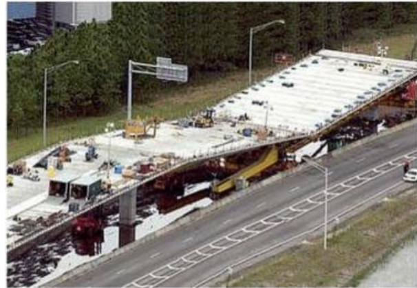
Fig. 12. The failed expressway viaduct after its pier had dropped into a void in the limestone beneath Tampa (photo: S. O'Rourke).
