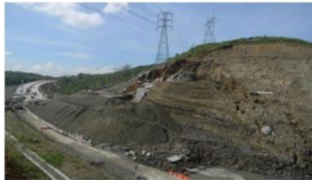
Figure 2.1.24 Slope Failure
