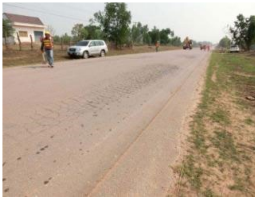
Figure 2.4.3 Pavement Damage due to Subgrade Deterioration on Laterite Base with Cement Stabilization (Laos)
