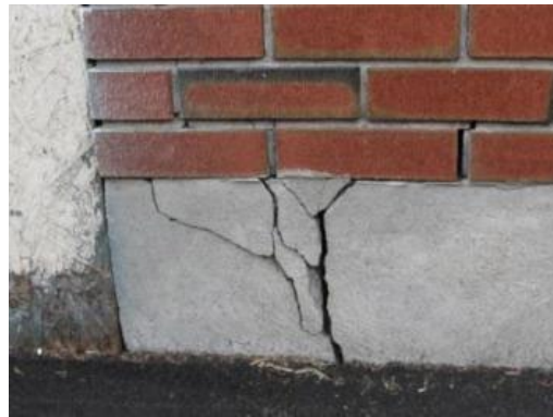
Figure 2.1.4 Pattern of damage to homes due to dome uplift.
