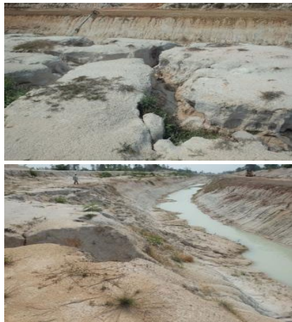
Figure 2.2.4 Typical Piping Hole
