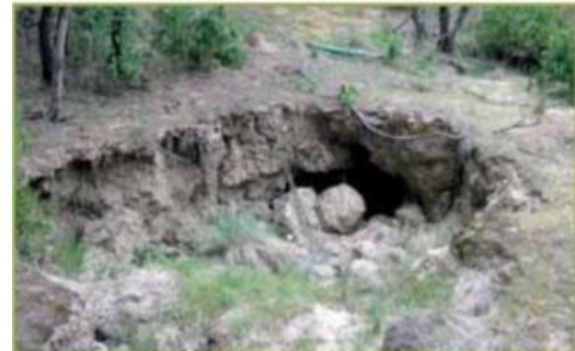
Figure 5. Piping failure or tunnel erosion in a dam constructed from soils derived from Permian mudstone. This dam is known to have failed on first filling. The image was taken from the dam floor.
