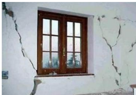
Figure 2.1.6 Example of damage to a house (cracks in the foundation)
