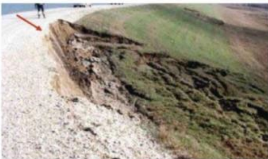
Figure 2.1.19 Damage to Embankment Slope (Indonesia)
