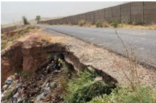
Figure 2.3.4 Settlement of loess and gully erosion
