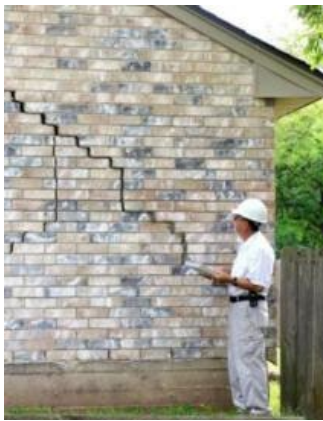
Figure 2.1.3 Dome-shaped uplifted deformation
