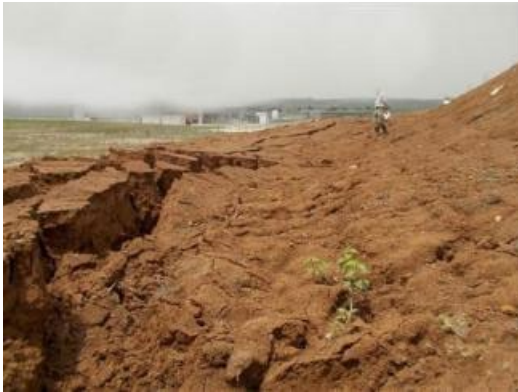
Figure 2.1.19 Damage to Embankment Slope (Indonesia)
