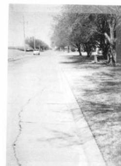
b. Looking north along east curb
