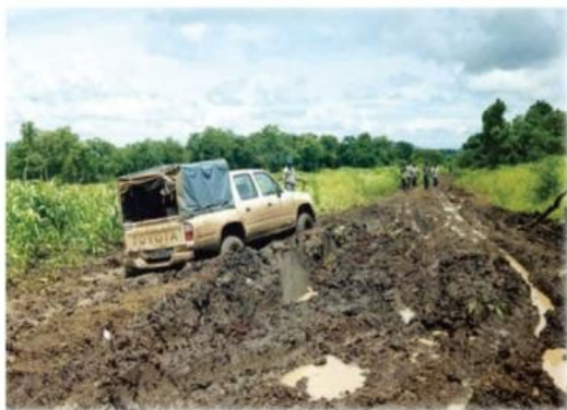
Figure 2-2: An entirely impassable section of an earth road (northwestern Ethiopia), due to soil expansiveness during rain periods leading to costly maintenance requirements.
