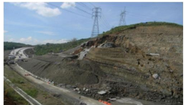
Figure 2 Slope failure at Toll Road Semarang-Bawen, Central Java, Indonesia (Himawan, 2011).
