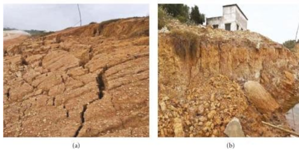
FIGURE 1: Cracking and collapse of expansive soil slopes.
