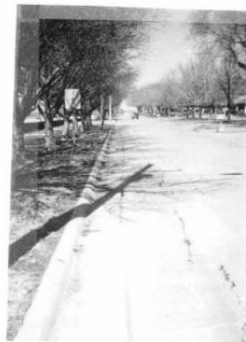
a. Looking north along west curb
