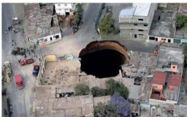
Fig. 10. The large dropout sinkhole in the suburbs of Guatemala City.
