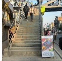
Installed near the pedestrian bridge near the bus stop
