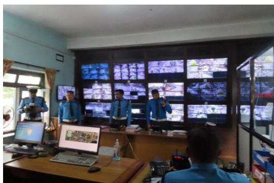
KVTPO Traffic Control Room
