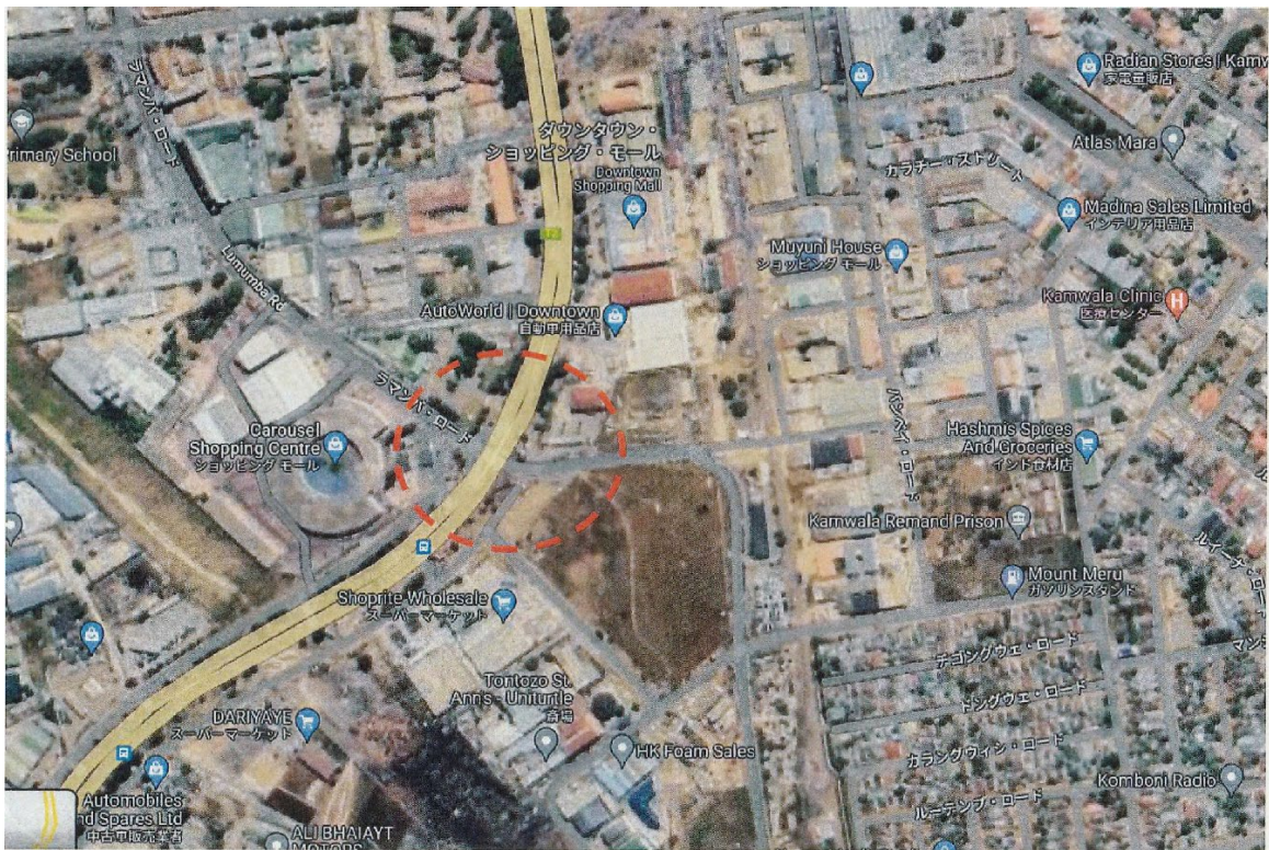
Flyover at intersection of Kafue Road and Lumumba Road (Tokyo way)
