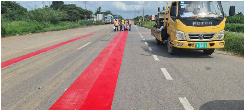
Figure 5.3.21 Installing Colored Road Markings on NR5 in Battambang Province
