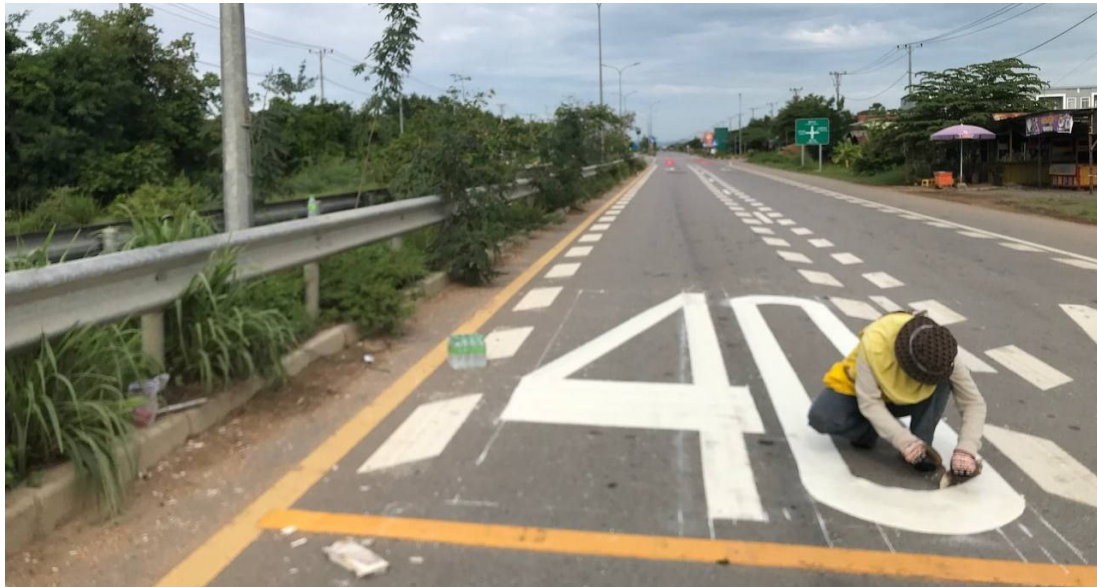
Figure 5.3.20 Installing 40 km/h Markings on NR5 in Battambang Province
