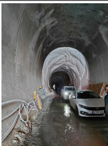
Figure 6-14 Connective Section of NATM and Open-Cut
