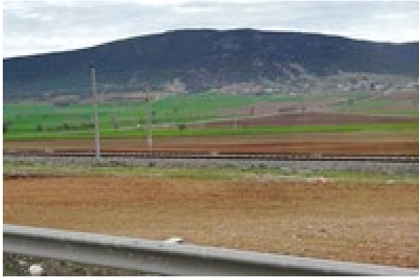
Figure 6-5 Section With Repaired Track
