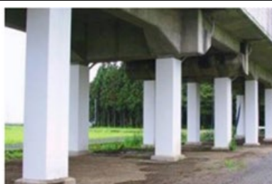
Reinforced Viaduct Pillars
