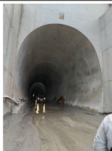
Figure 6-15 End of Open-Cut Tunnel
