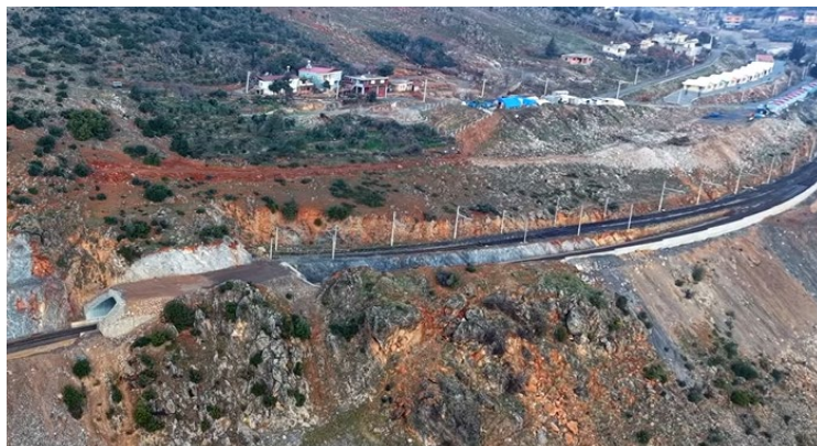
Figure 6-31 Retaining Wall for Landslide Countermeasures at Fevzipaşa Station
