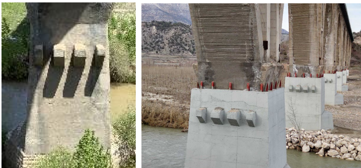
Figure 6-18 View of Pier C (Left: Before Restoration, Right: After Restoration)
