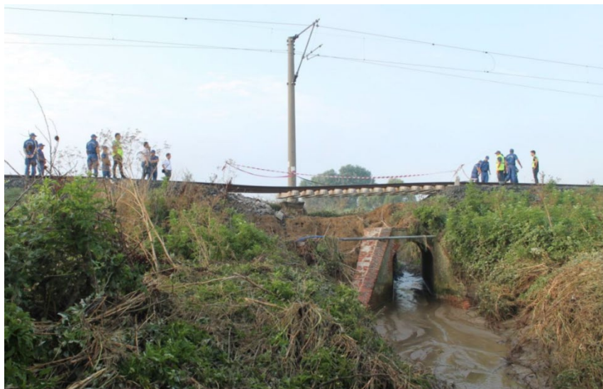
Figure 2-28 Culvert's Condition (Immediately After the Accident)
