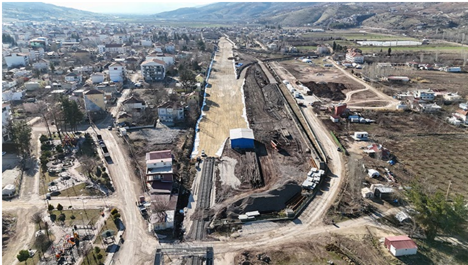
Figure 6-12 Replacement of Roadbed of Gölbaşı Station Area
