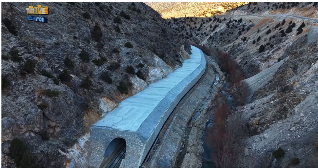
Figure 6-45 Completed Corrugated Tunnel
