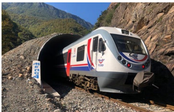
Figure 6-20 Rock-Fall Prevention Work Using Corrugated Plate Tunnel
