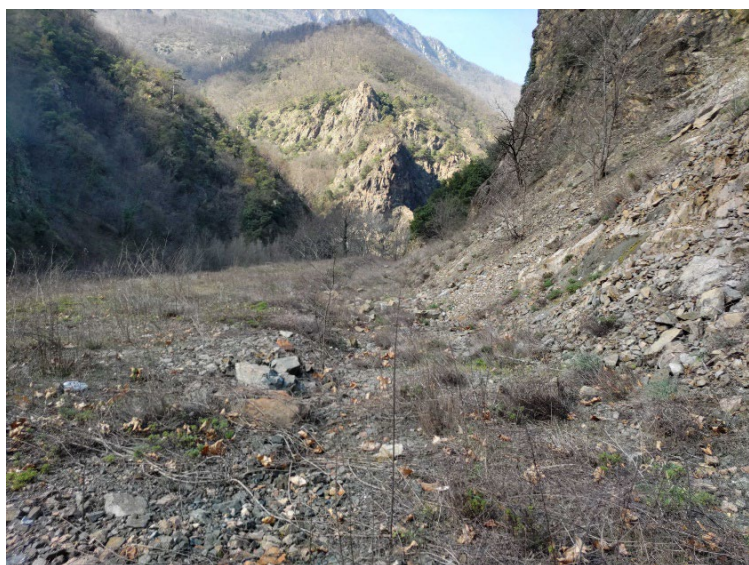
Figure 6-34 Gravel on Top of Corrugated Plate Tunnel Rock-Shelter Were Washed Away
