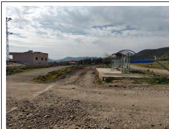
Figure 6-22 Situation Where Track Has Been Removed From 3 km Section
