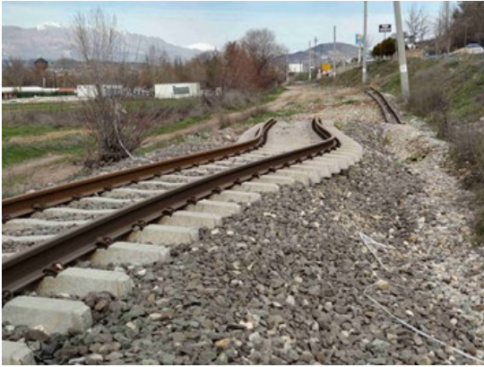
Figure 6-10 Large Deformed Track Near Gölbaşı Station
