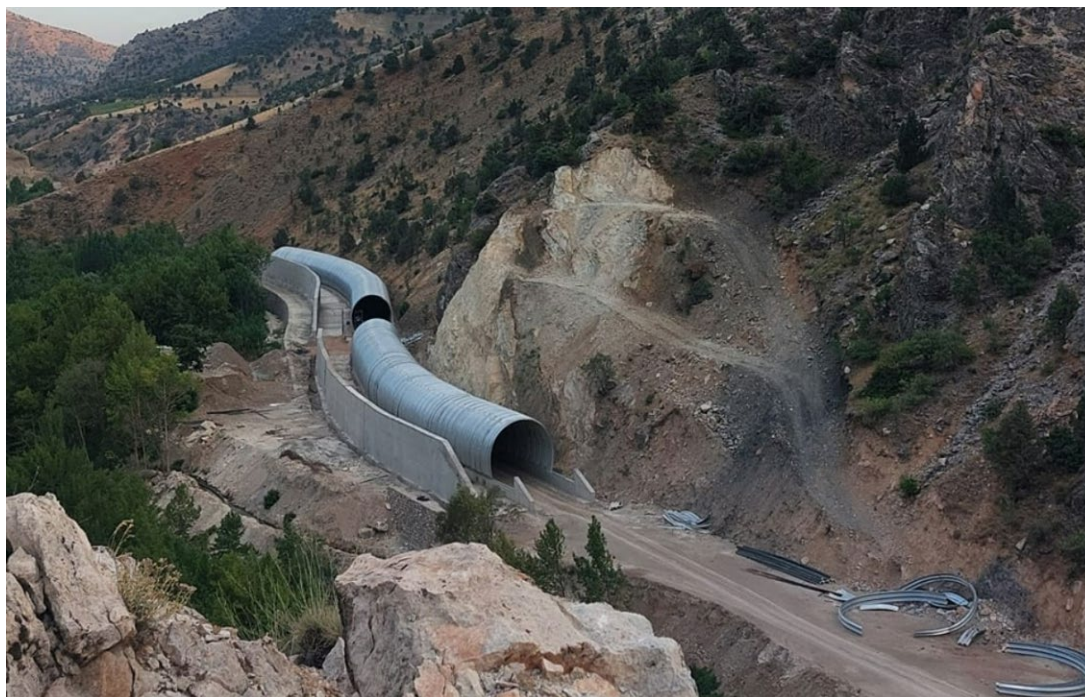
Figure 6-46 Corrugated Tunnel Under Construction
