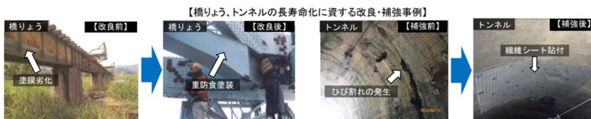
Measures against ageing facilities
