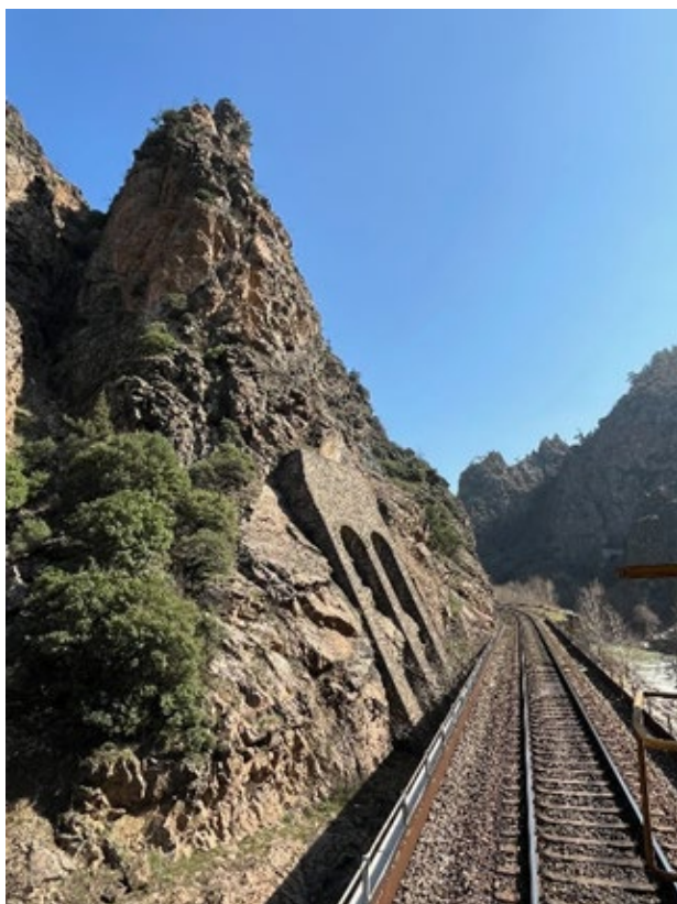
Figure 2-8 Rock Fall Protection Wall Constructed 100 Years Ago
