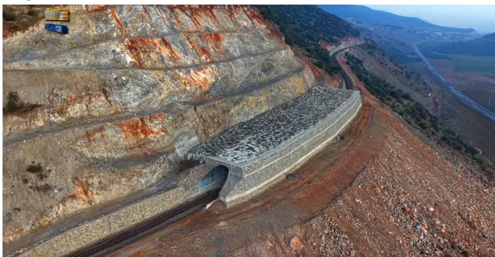
Figure 6-32 Rockfall Protection Using Corrugated Tunnel
