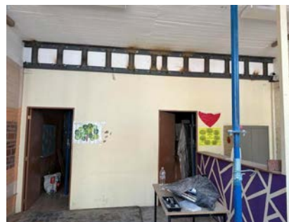
The site of seismic reinforcement work inside a classroom at this elementary school. The pillars and beams will be reinforced to improve earthquake resistance.
