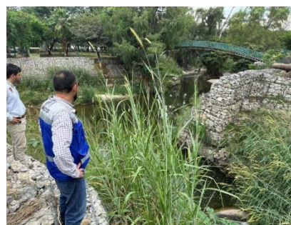
Confluence of the main Sabinal River and its tributary (the tributaries are more vulnerable to flooding than the main Sabinal River)
