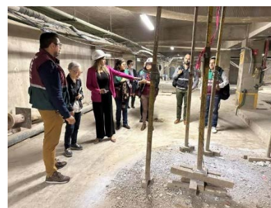
Talpan 550 apartment interior construction site. Piles and walls will be reinforced to improve seismic performance.
