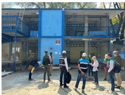
Earthquake-resistant construction site of Maestro Francisco César Morales elementary school damaged by the earthquake on September 19, 2017. Mexico City contributed 6 million pesos to the project, which is currently under construction with a 6-month construction period.
