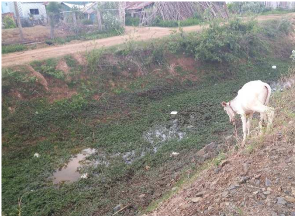
Photo: Irrigation Canal (Residential Property Encroaching on the ROW)
