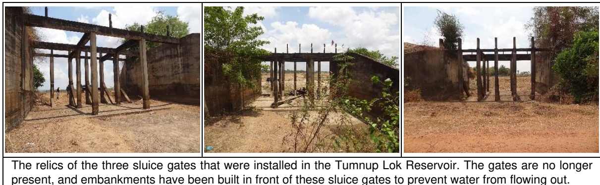
Figure 5.1.9 Current State of the Existing Sluice Gates Directly Connected to the Tumnap Lok Reservoir
