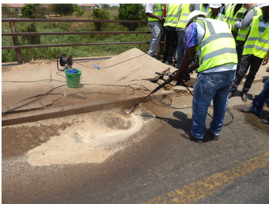
Photo 4-7 Cleaning of the Deck Slab and Its Drainage Inlet
