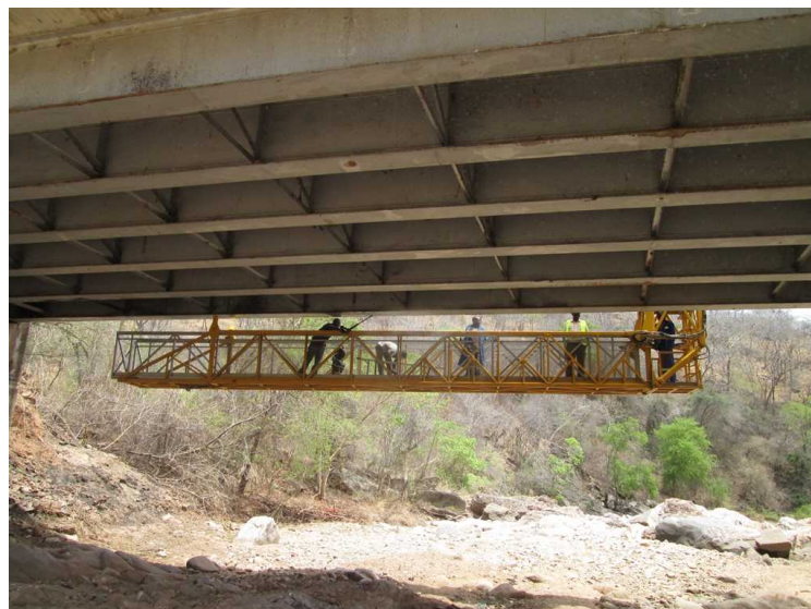
Photo 4-3 Cleaning of Steel Girder
