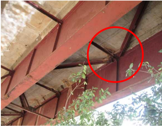
Photo 4-14 Corrosion occurred under the outlet of a drain pipe
