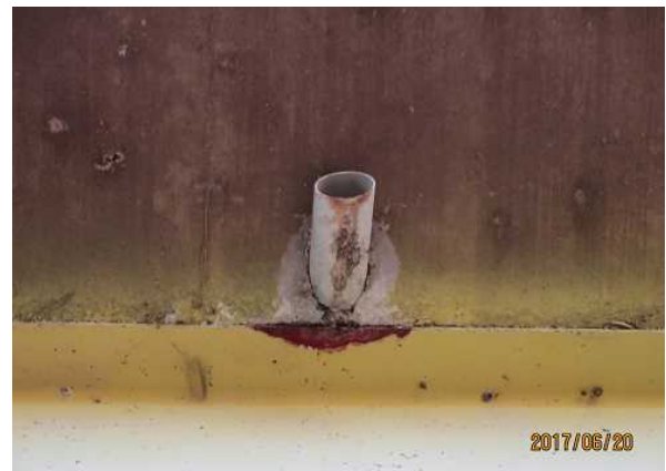
Photo 4-15 Deterioration at drain locations
