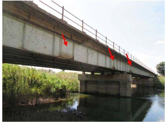
Photo 4-13 Deterioration at drain locations
