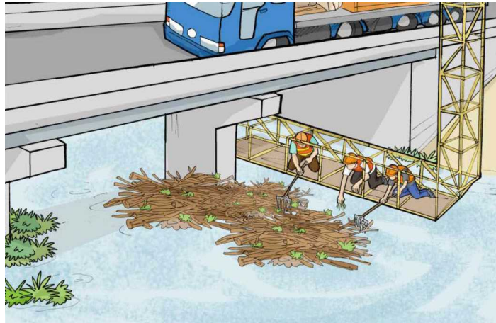
Figure 4-13 Removal of Drift Wood around Piers
