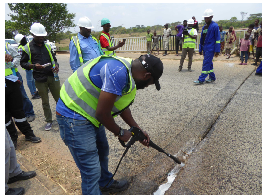
Photo 4-8 Cleaning expansion joint with high pressured water
