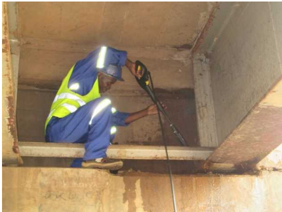
Photo 4-1 Cleaning of Bearing
