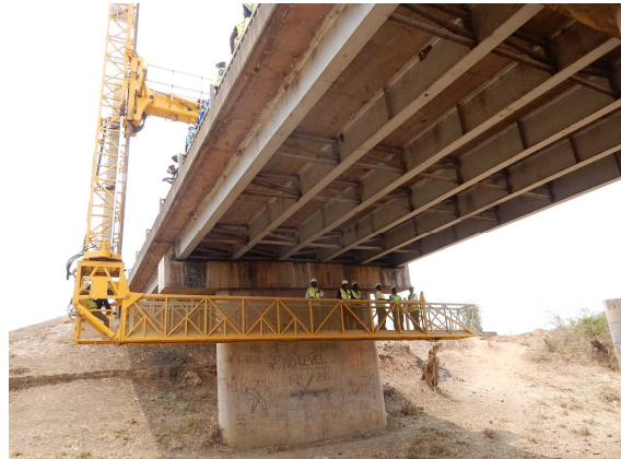
Photo 4-2 Cleaning using Inspection Vehicle
