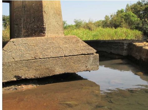
Photo 4-19 Exposed Pier Footing
