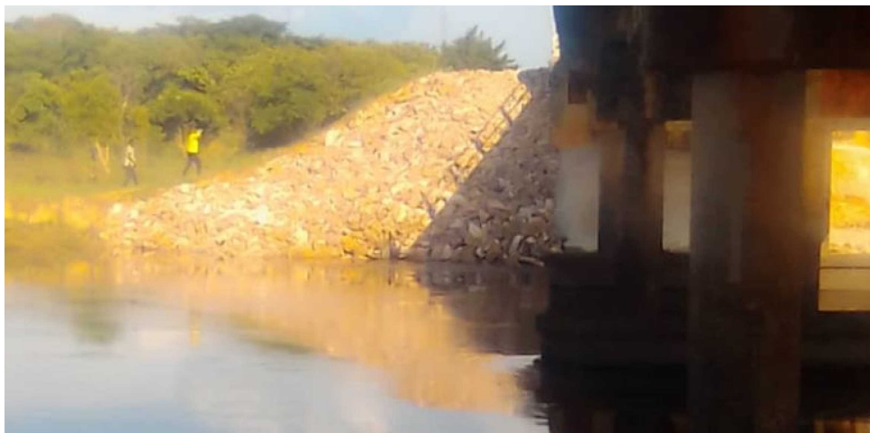
Photo 6-3 Repair around abutments
