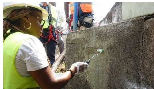
Practical training in repair work (Epoxy Coating)
