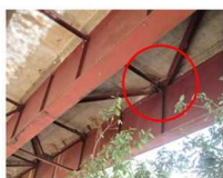
Photo 4-16 Corrosion occurred under the outlet of a drain pipe
