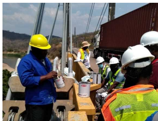
Touch-up Painting of Cable Anchorage
