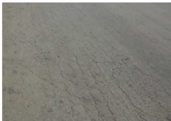
Longitudinal Cracks of Bridge Deck
