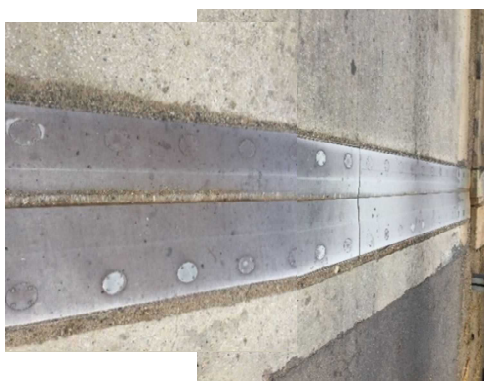
Lusaka Side Expansion Joint (Squeak and noise)
