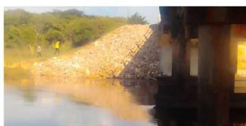
Photo 6-3 Repair around abutments
