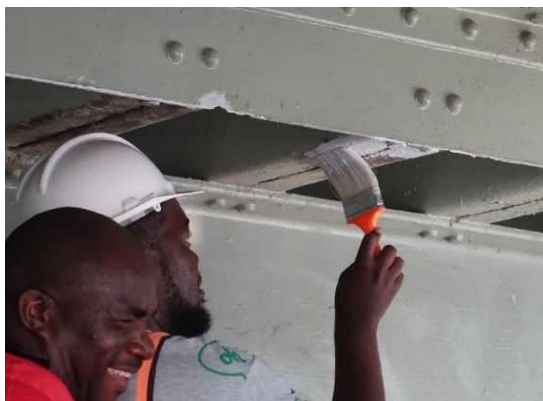
Practical training in repair work (Touch-up Painting)
