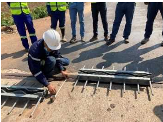
Expansion Joint Installation OJT at Rufunsa Bridge
