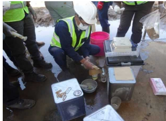
Injection Material Mixing OJT at Ruena Br.
