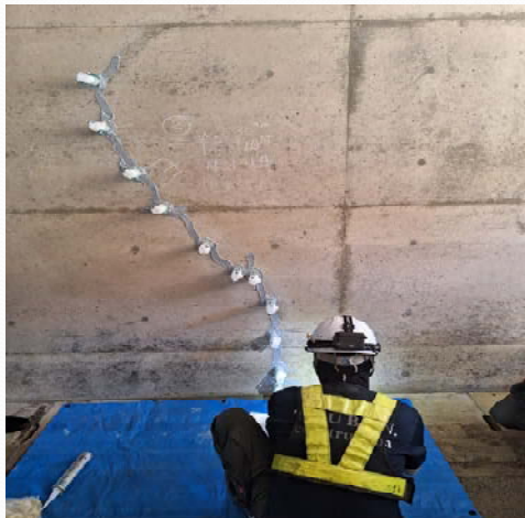
Concrete repair by sealing the cracks using epoxy injection method
