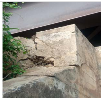
Abutment at Composite Bridge
