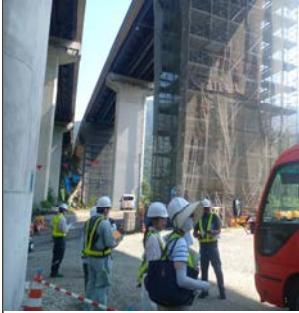
Reinforced Concrete (Kakinoshita Bridge)
