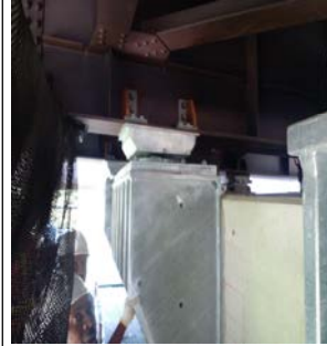
Horizontal Force- Dispersing Structure (Kakinoshita Bridge).
