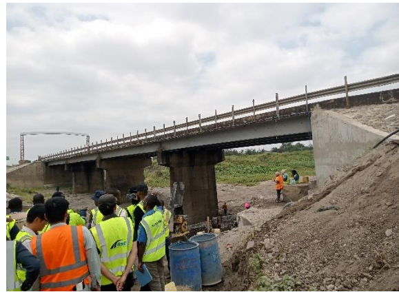
Inspection on scouring
