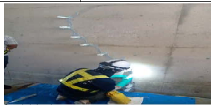
Crack Injection
