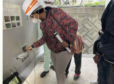
NDT Detection of cracks in Steel Members
