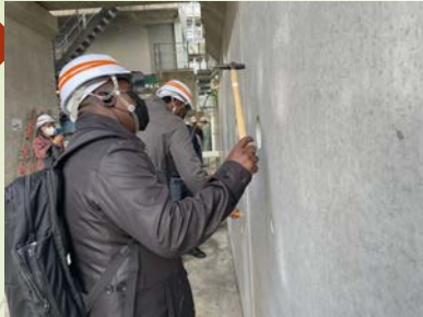
NDT for Concrete using the Hammer
