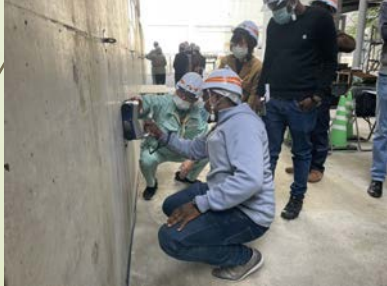
NDT Rebar Detection using Radar
