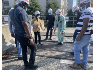
Demonstration of Waterproofing of Concrete Deck
