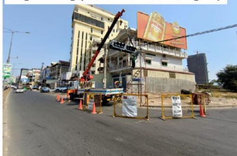
Engineering (Install new traffic signal)
