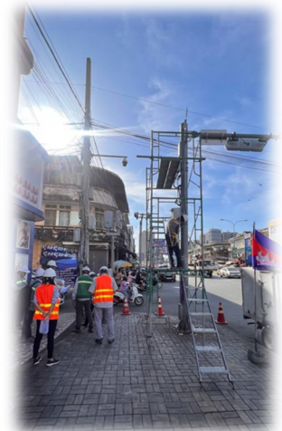
Installation and improvement of traffic signals through Piot Project
