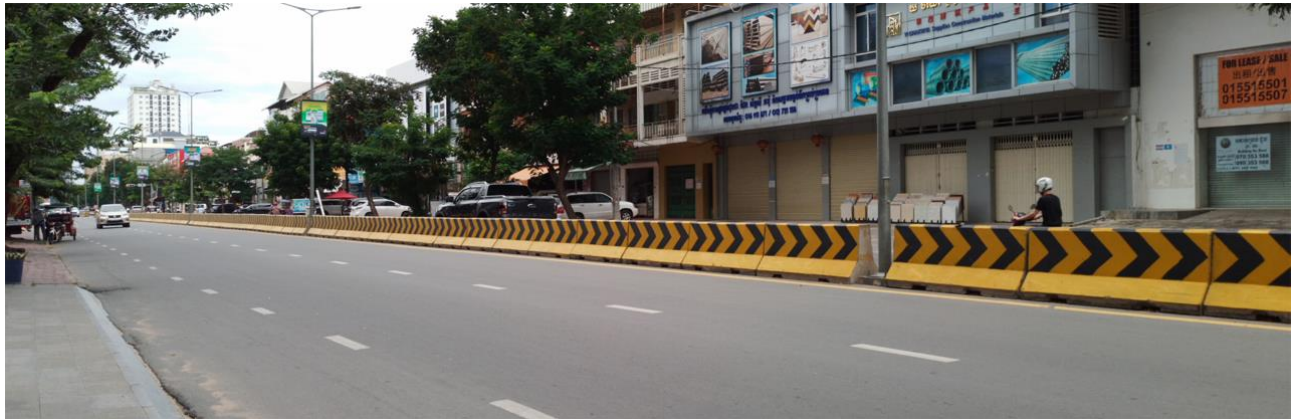
Figure 5.9 Concrete Barrier for Directional Separation of Traffic in Phnom Penh
