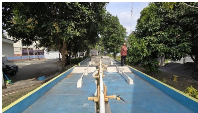
Figure 5-2 Panoramic view of outdoor hydraulic model experiment facility
