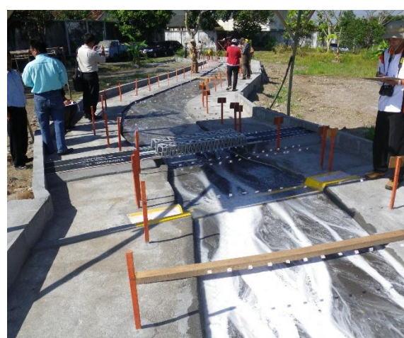
(Functional verification of a flood diversion channel designed for debris flow, 2011)
