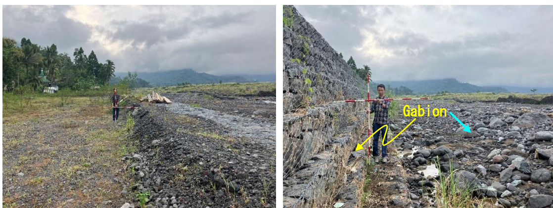
Figure 3-62 Current status of the Emergency Dike (May 2024)
