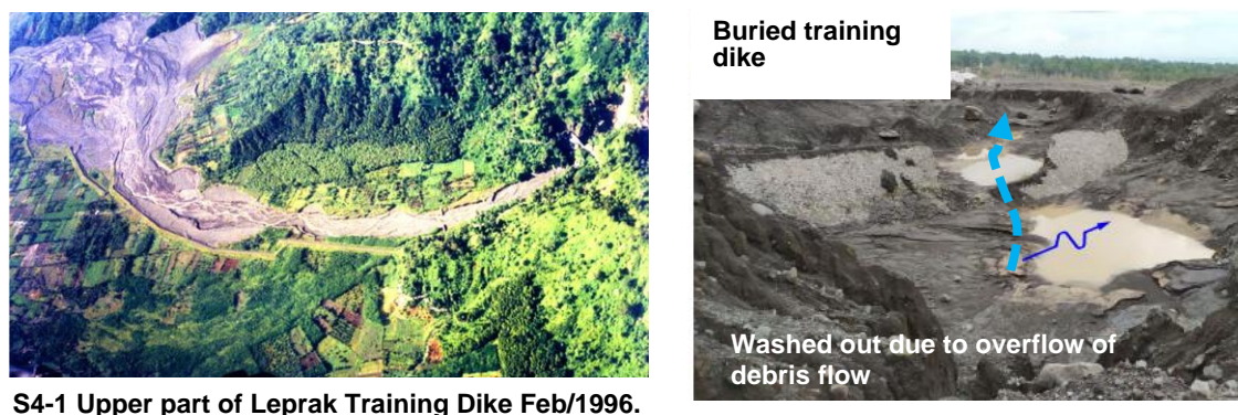
Figure 2-19 Overall view of Leprak training dike immediately after construction and dike eroded by debris flow (Dec 2021)
