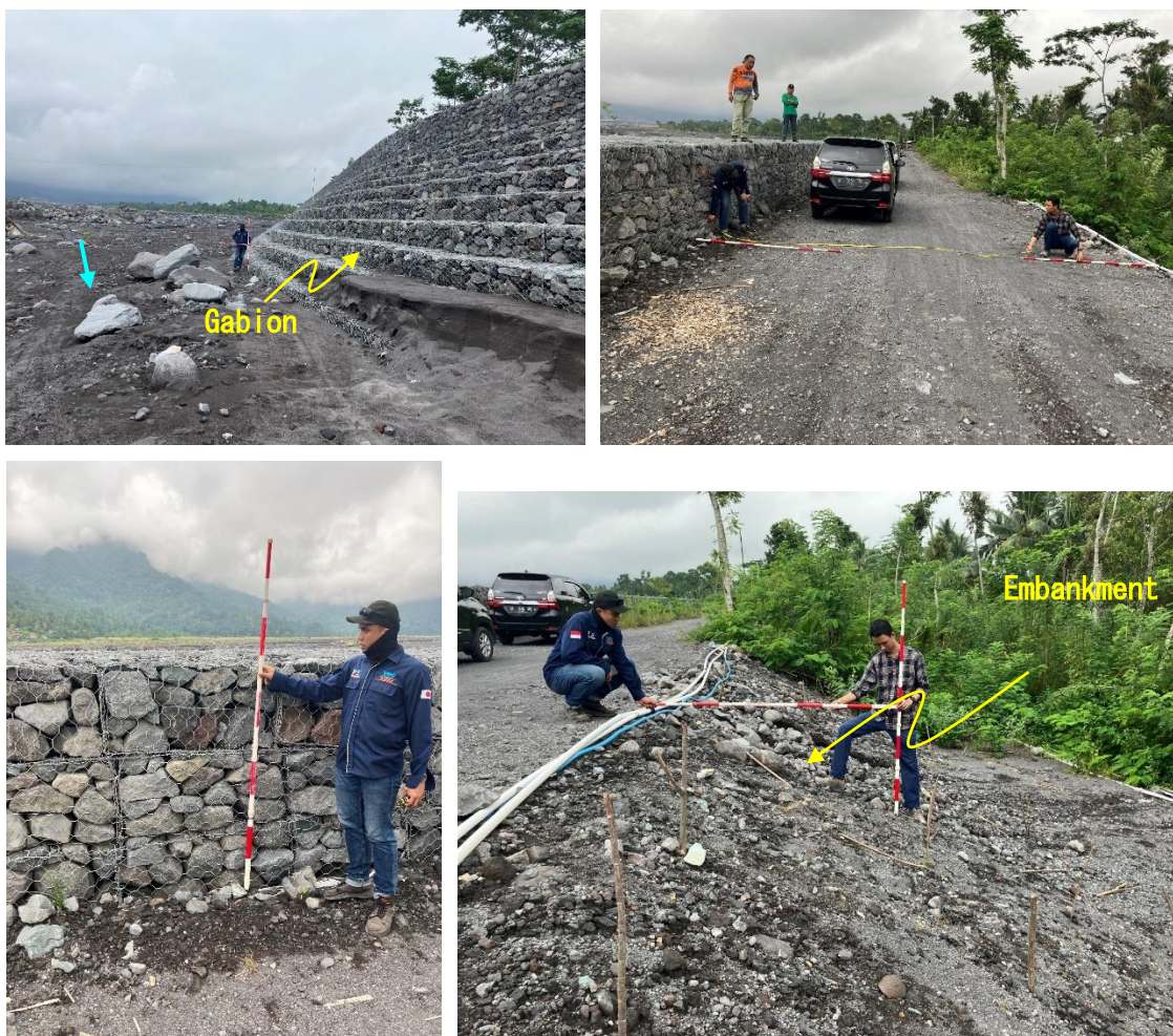
Figure 3-61 Current status of Tanggul Leprak XVII Kebondeli 2021 (May 2024)
