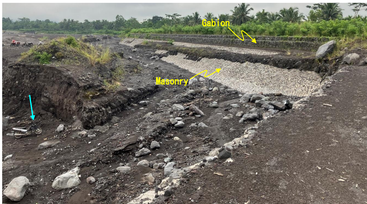
Figure 3-60 Current status of Tanggul Leprak II-D (May 2024)
