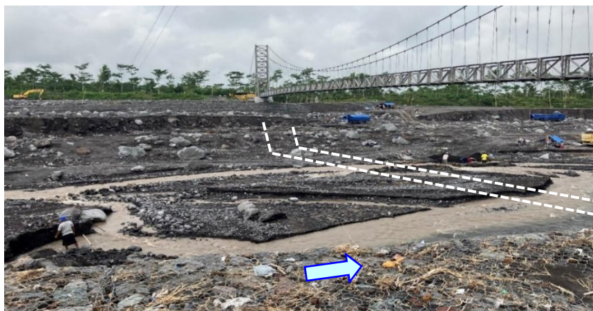
Figure 3-55 Damage to the left bank of KD Leprak 3 (May 2024)
