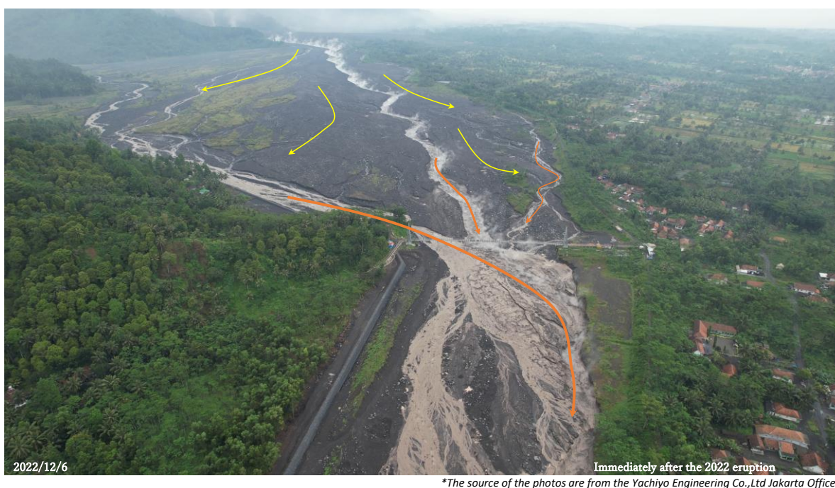
Figure 3-32 Condition of the midstream section (sand pocket section)
