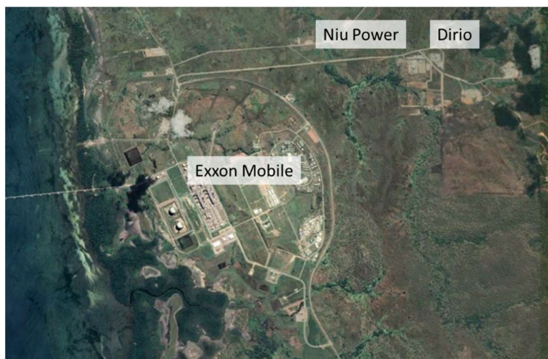
Fig1-2-2: IPPs connected to POM system
